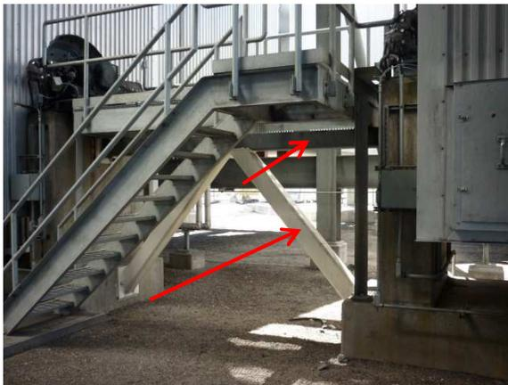
**Figure 3. ID Fan A & B, Outboard Pedestals, Steel Bracing Bolted to Each Pedestal.**
