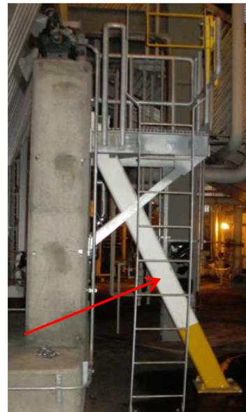
**Figure 4: ID Fan A Outboard Bearing Pedestal Single Brace 30 Deg Angle.**
