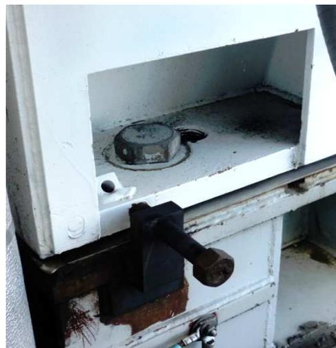
**Figure 8. ID Fan A & B Motor Hold Down Bolts Used Tapped Holes in Fabricated Steel Base.**
