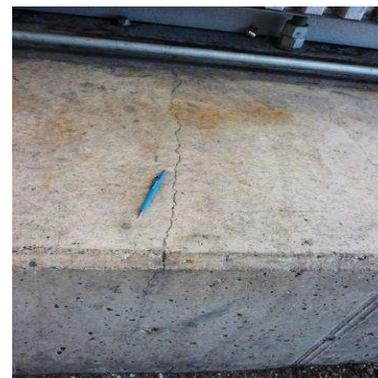
**Figure 5. ID Fan A Foundation Crack.**
