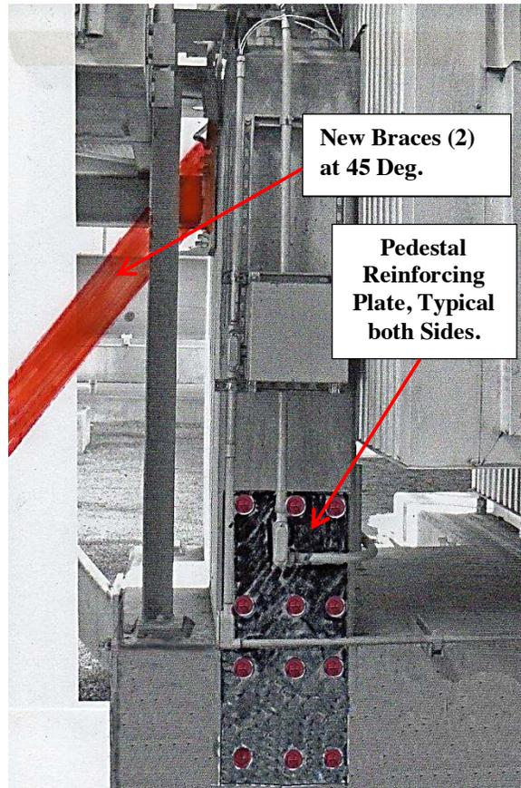
**Figure 35. Remove Existing Steel Braces and Install Two Braces at 45 Deg. Bolt Plate to Each Side of Pedestal & Concrete Foundation.**
