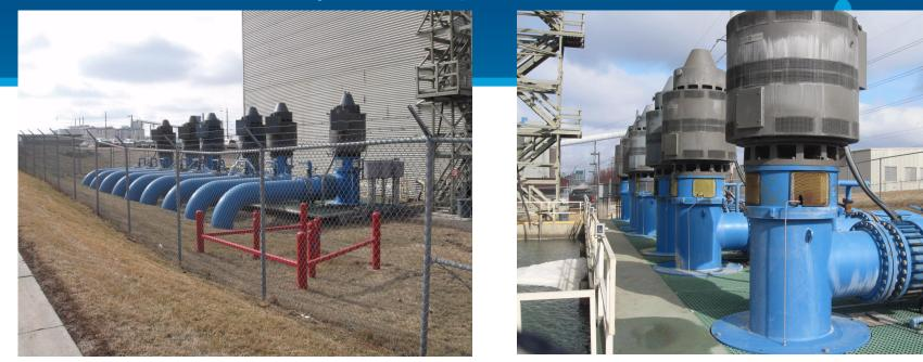
Vertical pumps servicing a cooling tower at a co-generation facility were experiencing premature bearing and seal failures. The pump array consisted of six 1,000 hp units, supported on a common flexible steel framing system that spanned the sump pit. Provisions (pipe stubs) were provided for future expansion to include three additional pumps, for an eventual total of nine pumps. The operating speed of the pumps was 900 rpm (15.0 Hz).
