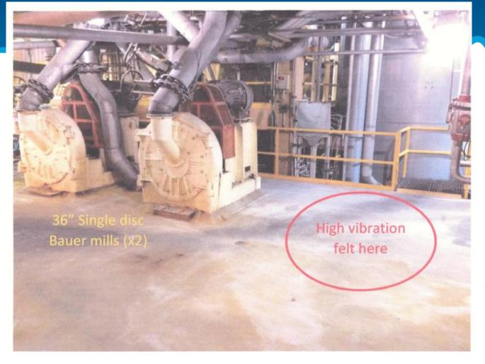
Milling Machine on Concrete Slab supported by Structural Steel Framing. Machine Speed = 890 rpm = 14.83 Hz Floor Vibration Nuisance
