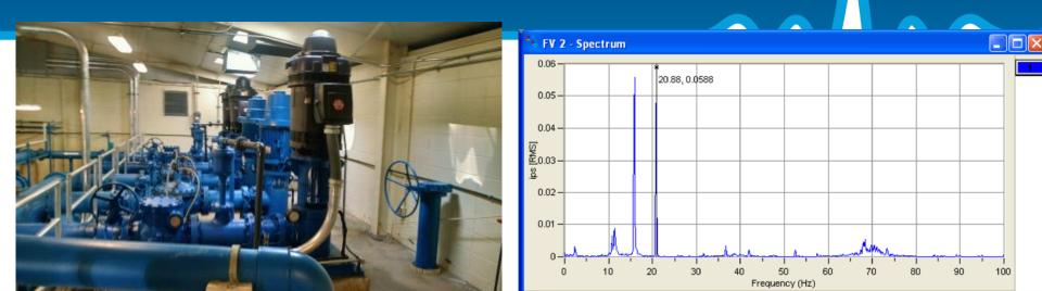
1800 rpm Pump Operates with VFD Control. At low flow (speed) settings, check valve not completely open. A rotating stall condition initiates. Vibration @ subharmonic frequency (~16 Hz) as well as operating speed (1250 rpm ~ 20.88 Hz).
