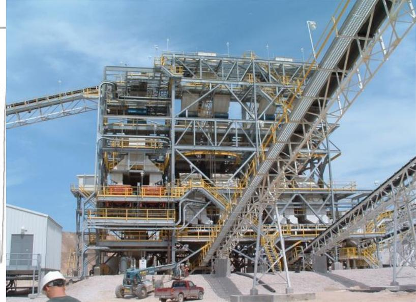
Structural vibration was dominated by response at 4.3 Hz, reaching magnitudes of 2.4 ips with the machine only lightly loaded.
