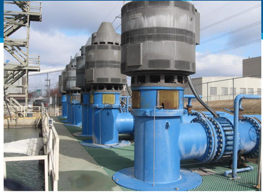
Vertical pumps servicing a cooling tower at a co-generation facility were experiencing premature bearing and seal failures. The pump array consisted of six 1,000 hp units, supported on a common flexible steel framing system that spanned the sump pit. Provisions (pipe stubs) were provided for future expansion to include three additional pumps, for an eventual total of nine pumps. The operating speed of the pumps was 900 rpm (15.0 Hz).
