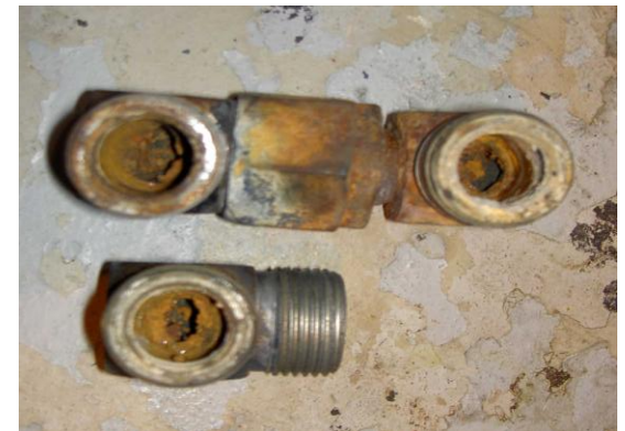
Cooling Tubes Plugged
