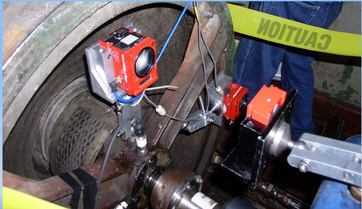
Figure 34. Permalign Setup on Blower and Motor. Ref 7
