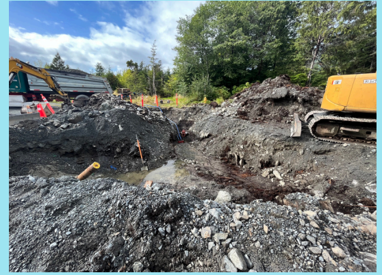
The site is now connected to sewage and water infrastructure.
