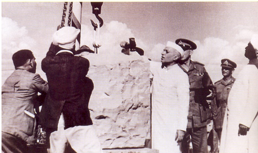
"A Monument in the Making" – Pt Nehru, the Hon'ble PM of India, laying the foundation stone at Khadakwasla on 06 Oct 1949
