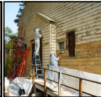
Lead Paint Abatement
