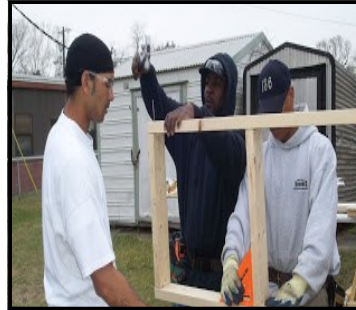
Basic Construction Skills
