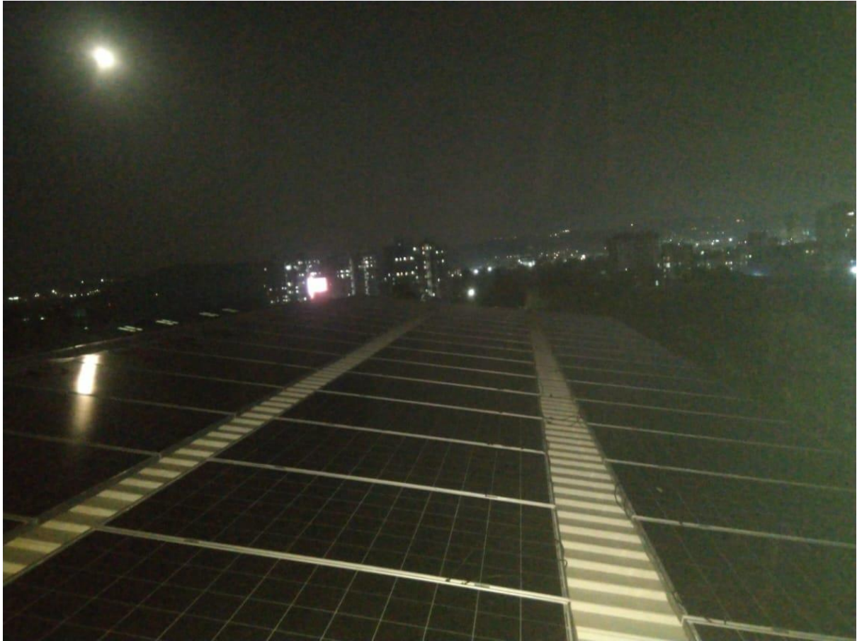
60 KW Rooftop Composite System-Pioneer Pvt Limited, Pirangut (Photo-1)
