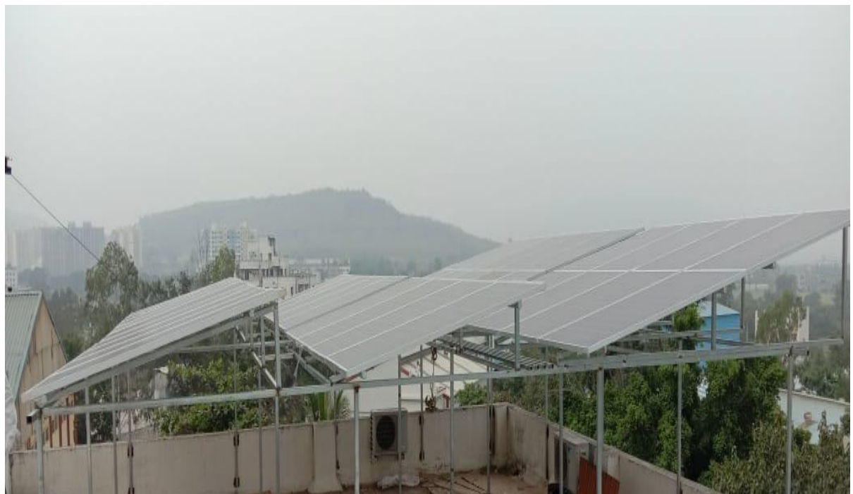
60 KW Rooftop Composite System-Pioneer Pvt Limited, Pirangut (Photo-2)
