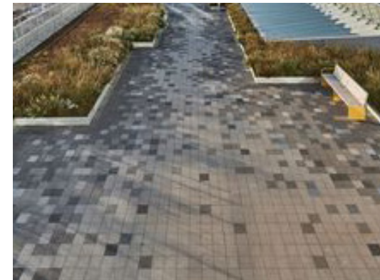
Decorative permeable cement concrete paving
