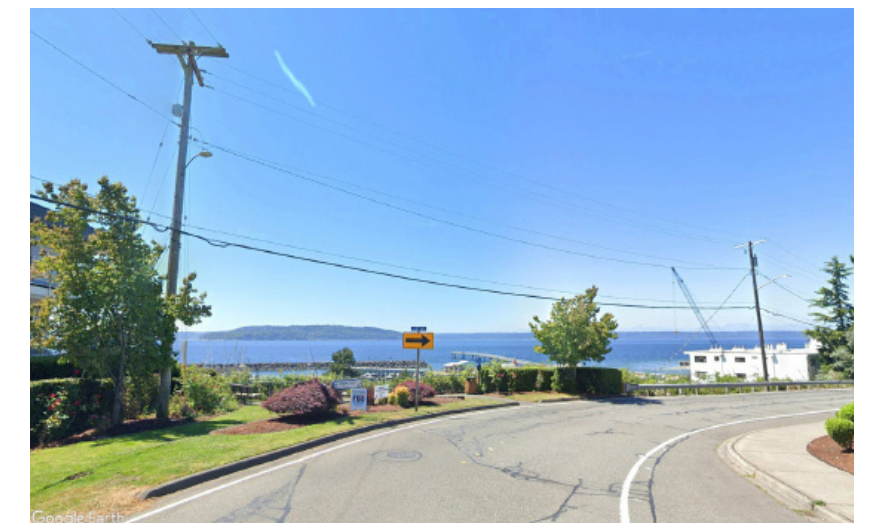
Overhead utility lines at Overlook I Park
