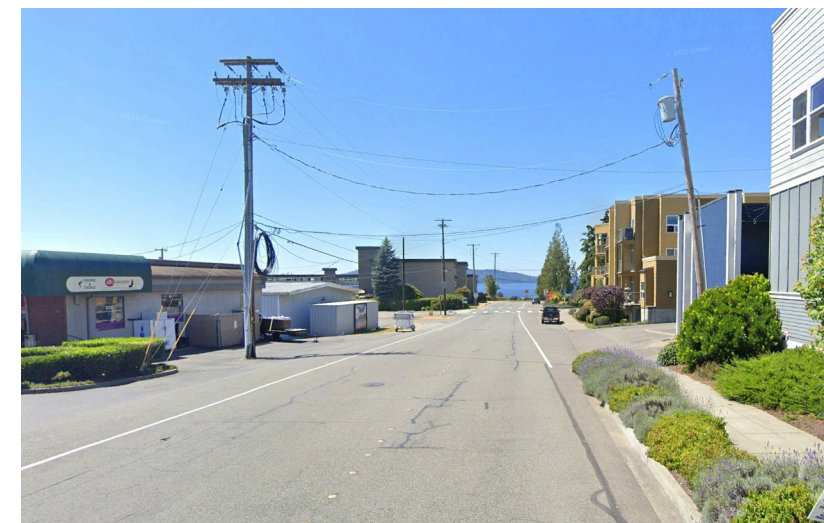
Overhead utility lines just east of S 223rd St and 7th Ave S intersection
