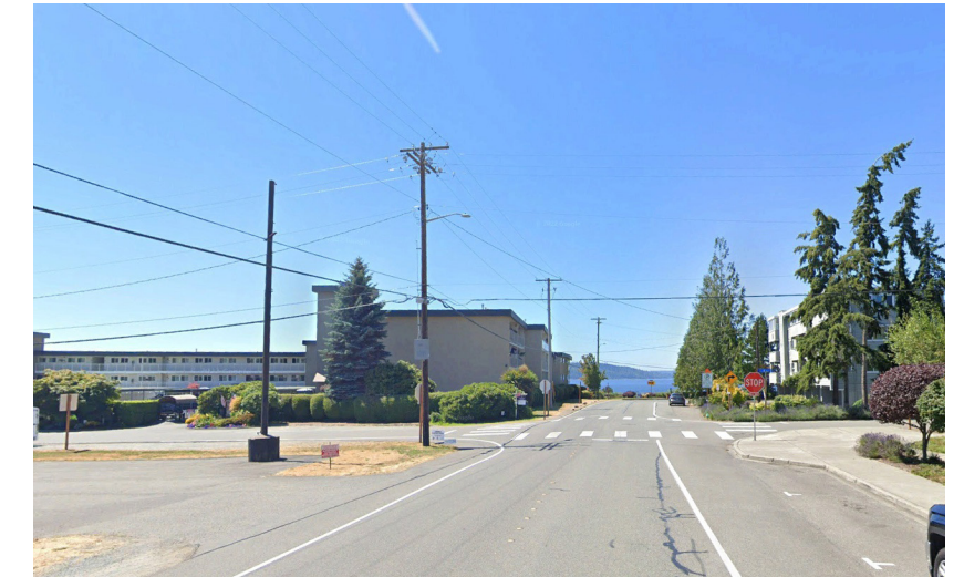
Overhead utility lines at S 223rd St and 6th Ave S intersection
