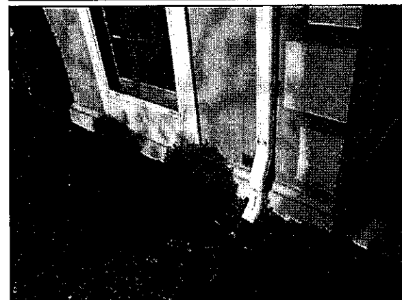
Photo #30. Downspout at Community Center discharges at the building foundation.
