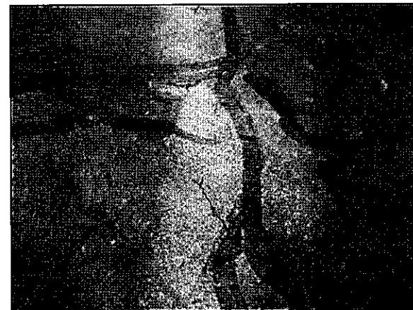
Photo #138. Depressed and alligatored asphalt pavement at the Community Center parking area.
