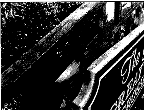
Photo #83. Typical failing paint system on decorative metal at entrance monument.
