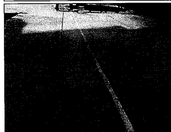
Photo #48. Typical cracks in the pool deck.
