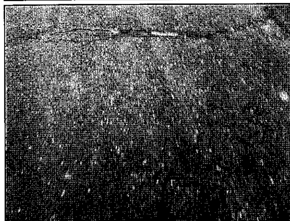
Photo #107. Cracks in Hunter Gate Way pipestem.
