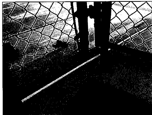
Photo #70. Defective sockets and crack in pool deck.
