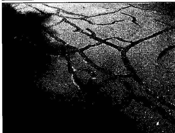
Photo #101. Large open cracks in the asphalt pavement at the townhouses.
