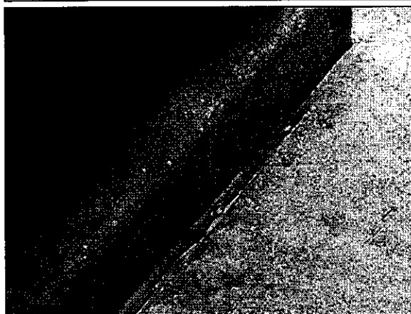
Photo #77. Failed sealant between pool deck and stoop.
