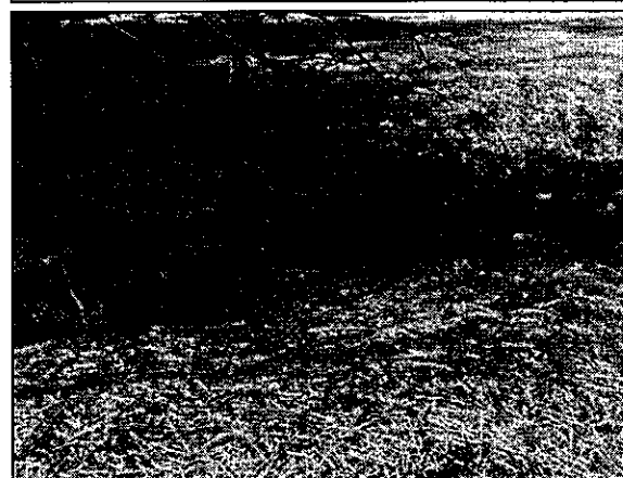
Photo #150. Spillway is not reinforced and will be easily damaged by erosion.
