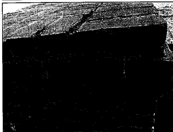
Photo #89. Typical entrance monument masonry construction in need of tuckpointing.
