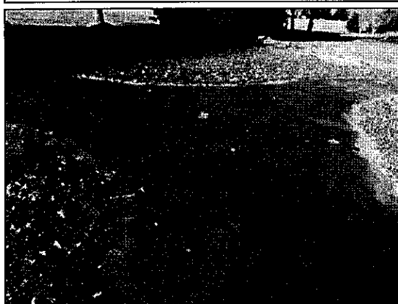
Photo #95. Large open cracks in the asphalt pavement in the open space southeast of the townhouses.
