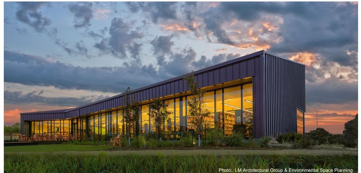
Photo: LM Architectural Group & Environmental Space Planning
