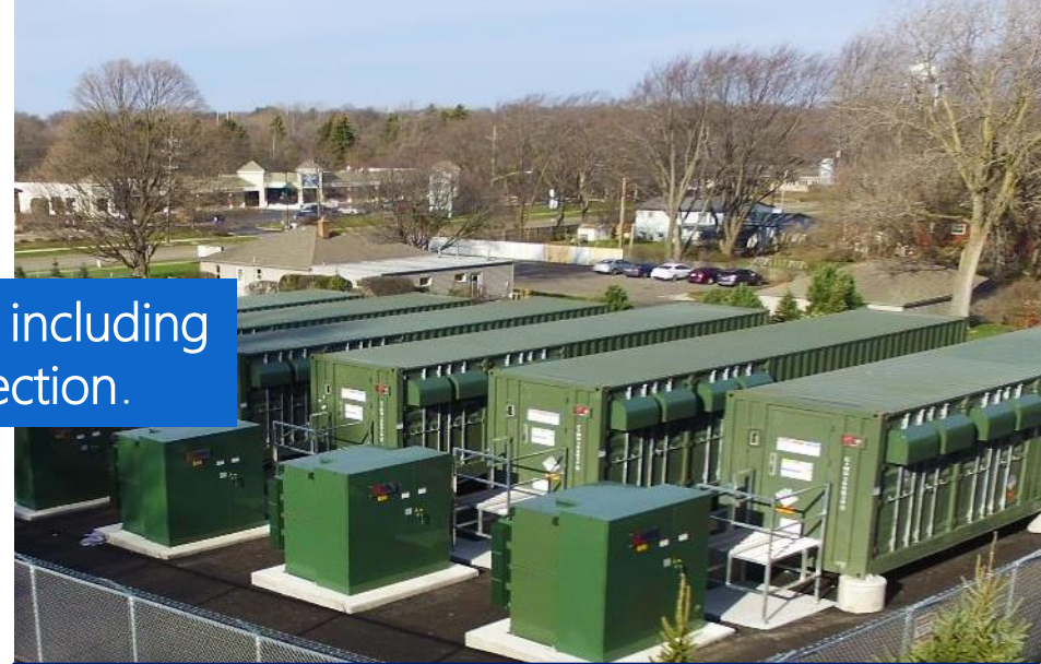
Battery Energy Storage Systems (BESS)
