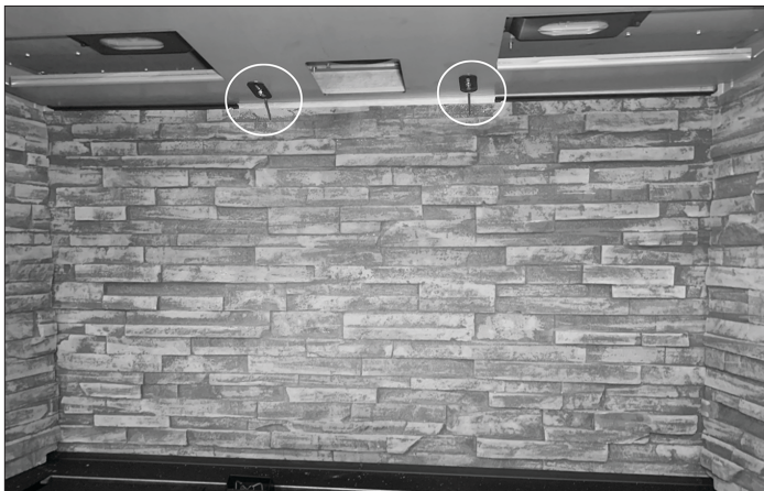
Figure 8.3, Back Refractory Panel Installed
