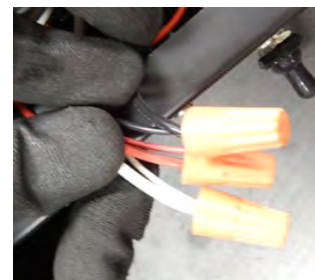
Figure 39 Connecting the wires
