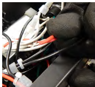
Figure 38 Connecting the wires
