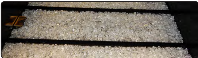
Figure 7.b Completed fireglass installation
