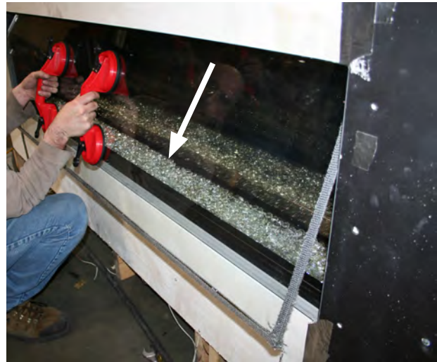
Figure 2 Sec.8 Window Removal (using glass lifting tools).
