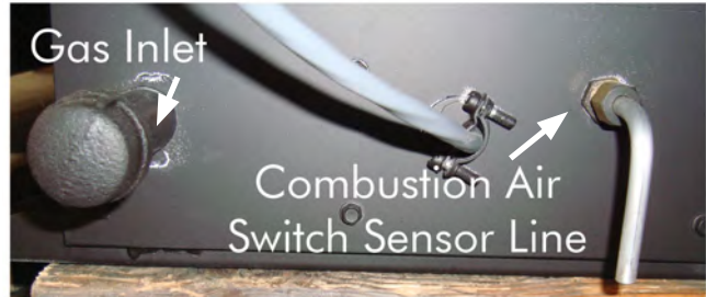
Figure 2 Sec.6 Identifying the Gas Inlet and Combustion Air Switch Sensor Line
