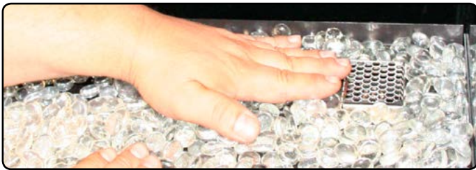
Figure 11.d spreading out firestones
