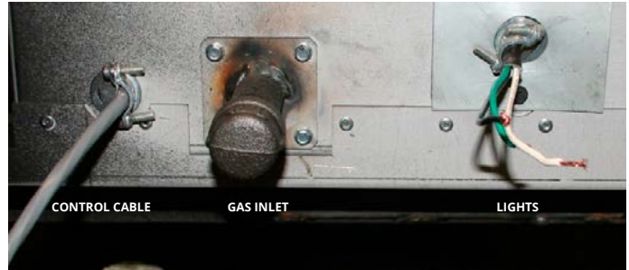
Figure 9.b.b Identifying the Gas Inlet
