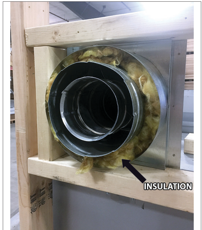
Figure 7.4, Pass-through with square rigid frame
