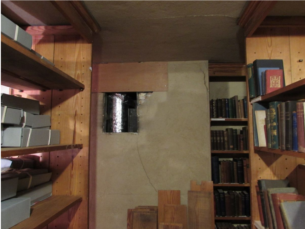
Photo #83 – Opening in HVAC Chase (3 rd Floor Stack Room)
