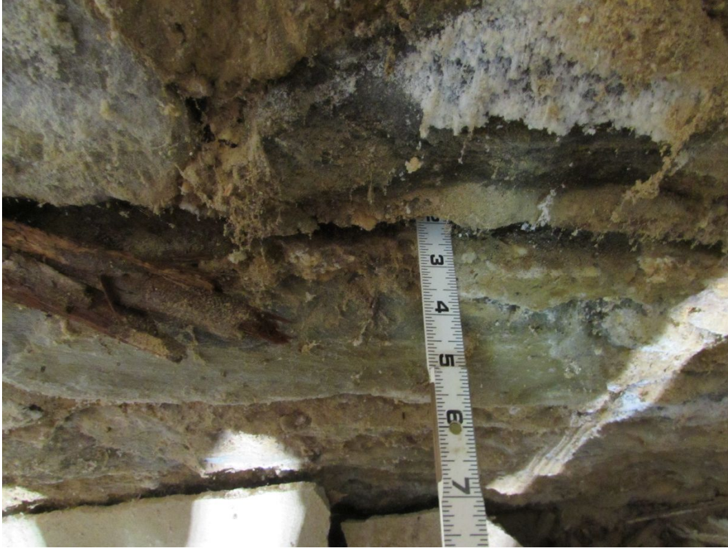
Photo #8 – Decayed wood nailing joint in foundation wall of photo #6
