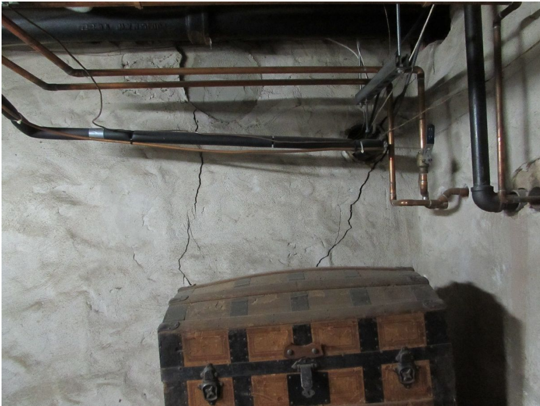
Photo #13 – Vertical and diagonal cracking noted in photo #12 above
