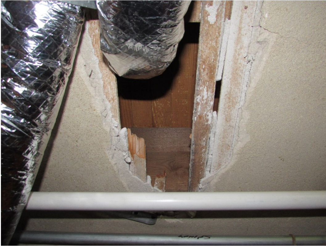
Photo #44 – Opening in plaster ceiling
