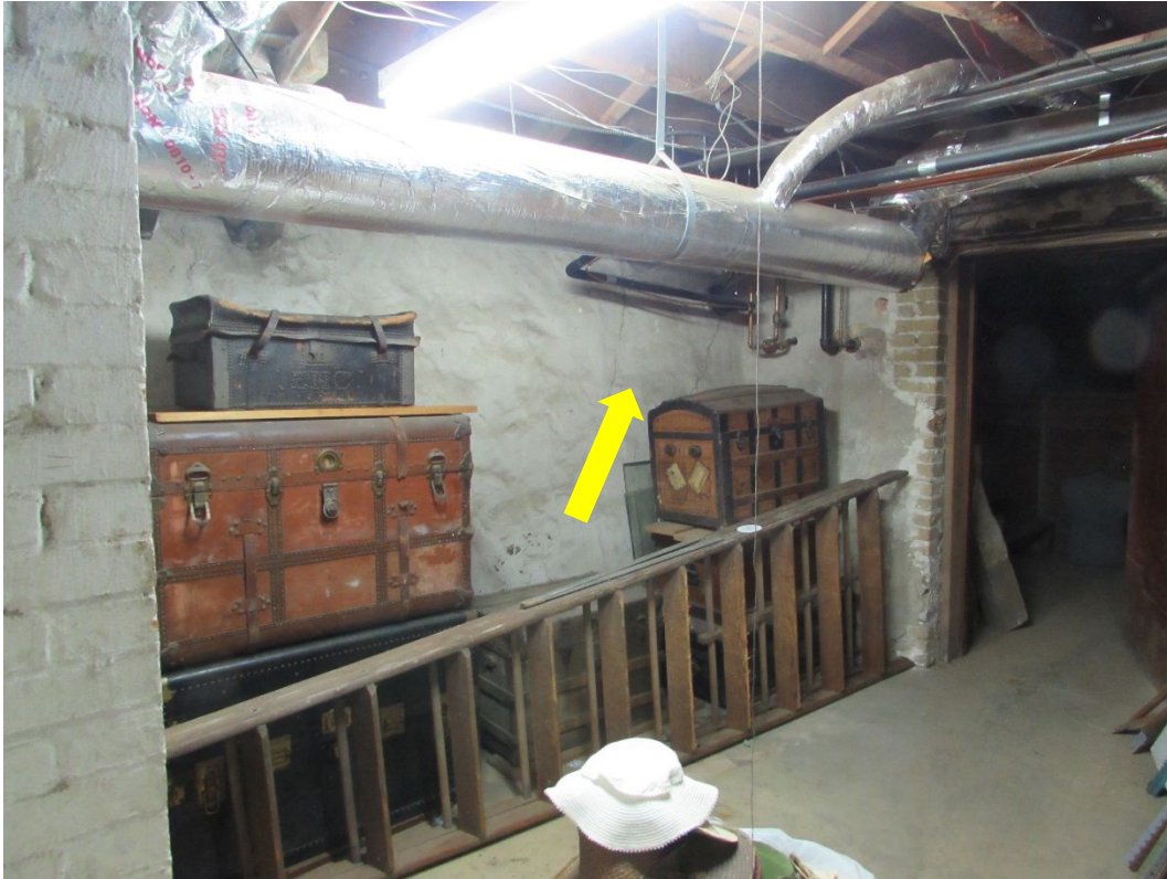
Photo #12 – Interior foundation wall common to workshop, location of cracking noted
