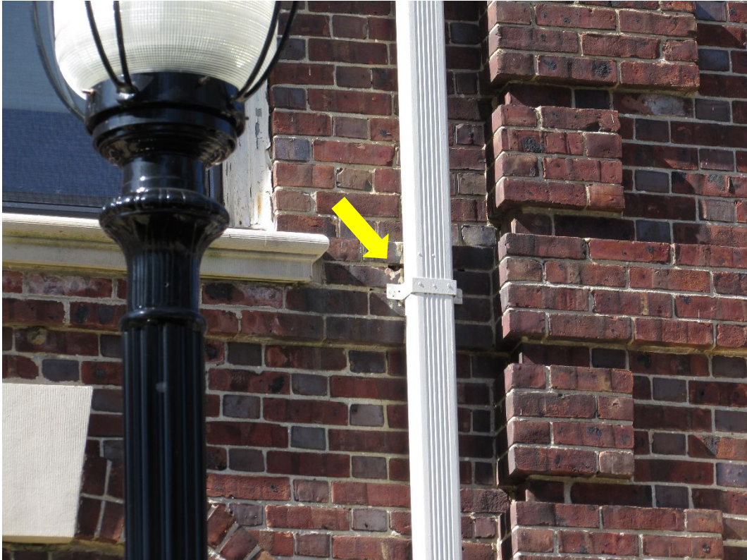
Photo #94 – Open mortar joint
