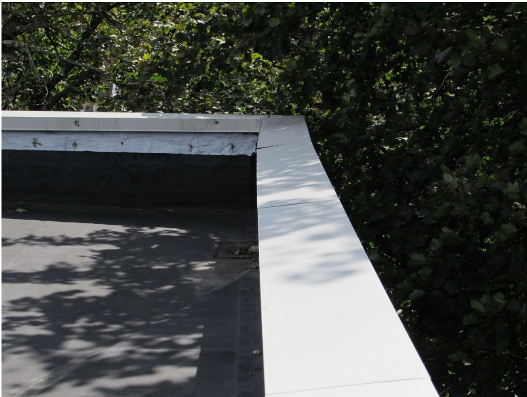
Photo #115 – Rear parapet wall leaning inward
