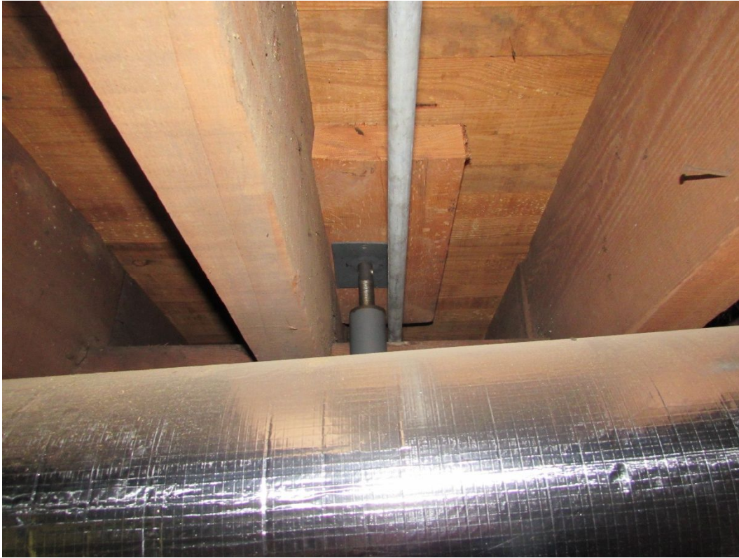
Photo #28 – Deformed cap plate of column depicted in photo #27
