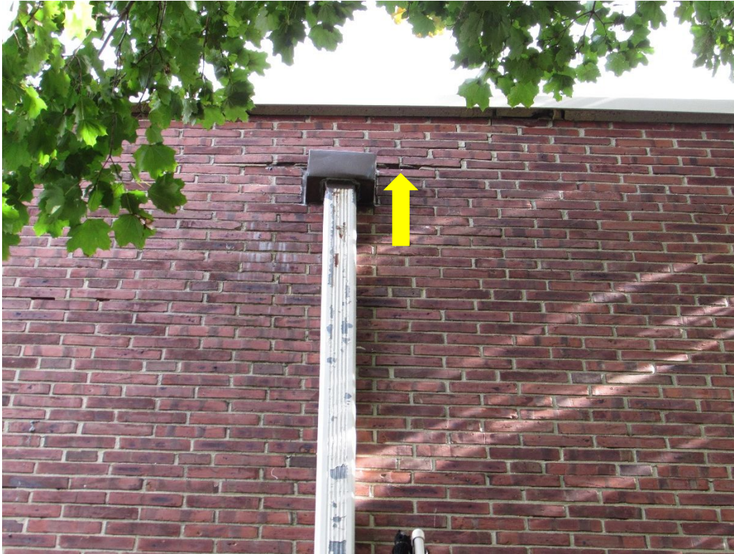
Photo #108 – Appearance of minor lateral displacement at roof scupper
