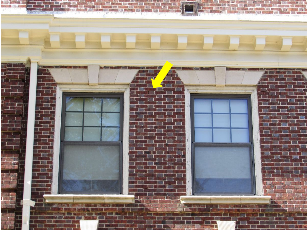
Photo #92 – Open mortar joint
