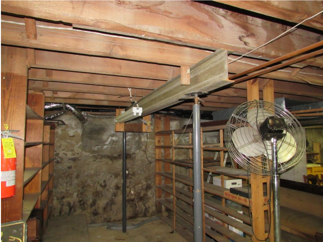
Photo #38 – Beam and columns installed to support cracked floor joists
