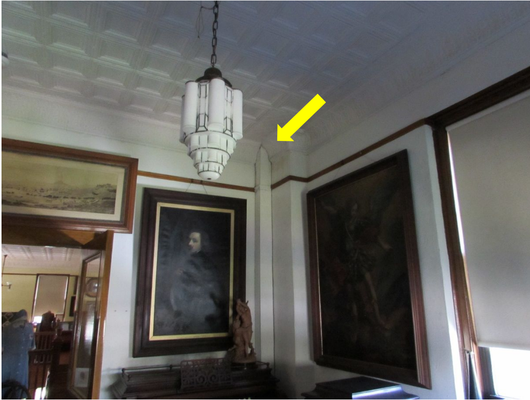
Photo #70 – Water infiltration at 1933 addition
