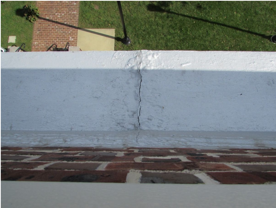
Photo #116 – Looking down from roof at open seam in perimeter trim
