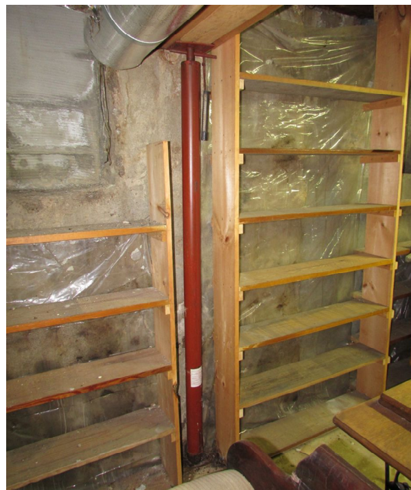
Photo #25 – Corroded steel column
