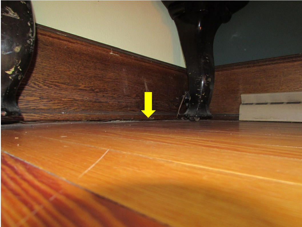
Photo #54 – Gap between wall trim and floor depicting floor movement
