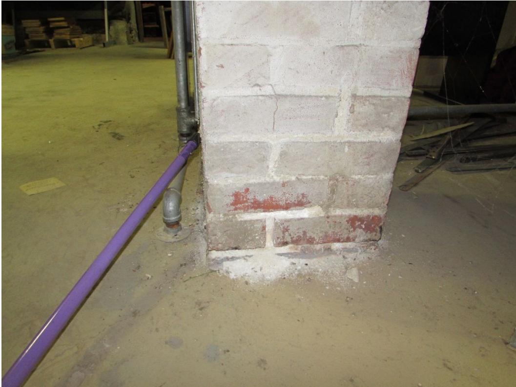
Photo #23 – Deteriorated mortar at base of pier
