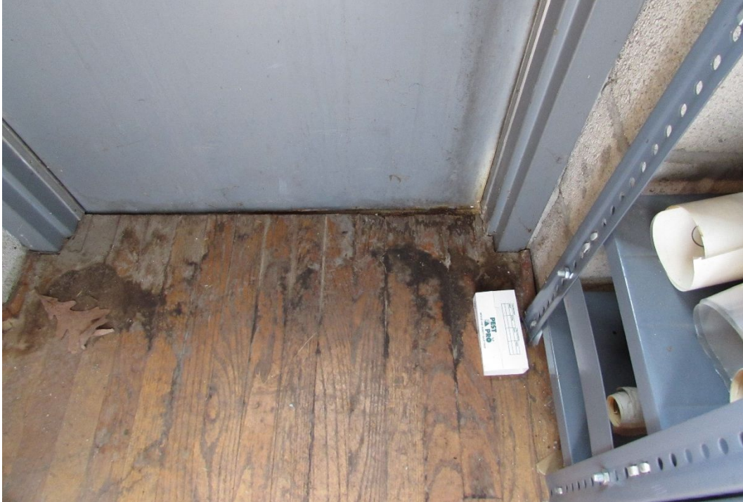
Photo #86 – Water intrusion at emergency exit
