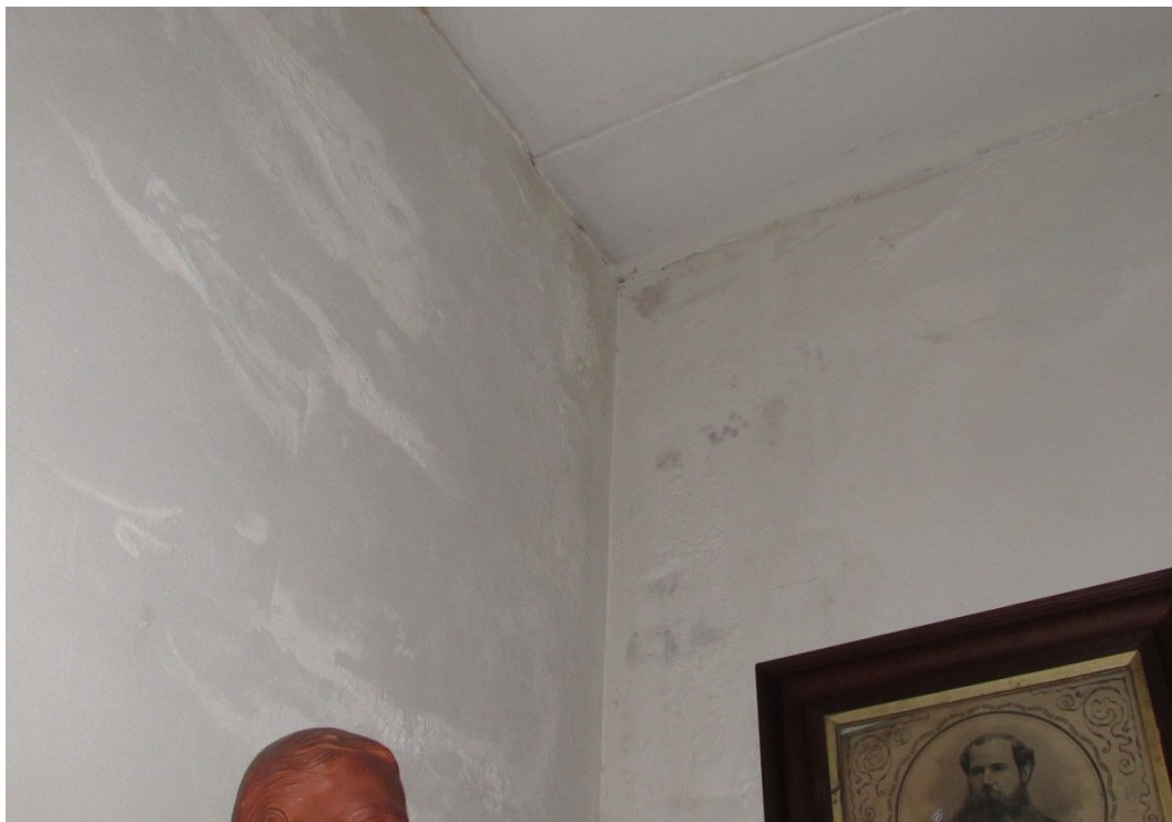
Photo #75 – Water infiltration (paint blisters and staining) at Civil War Gallery
