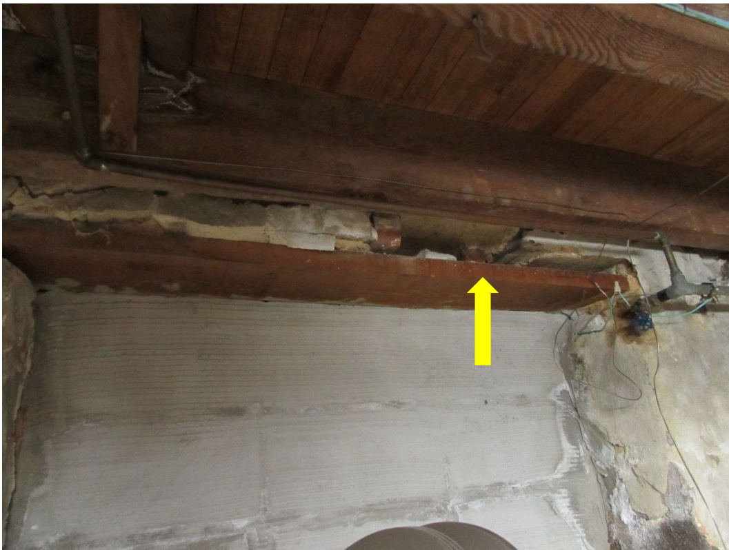
Photo #10 – Poorly infilled window opening, note wood header with loose brick above
