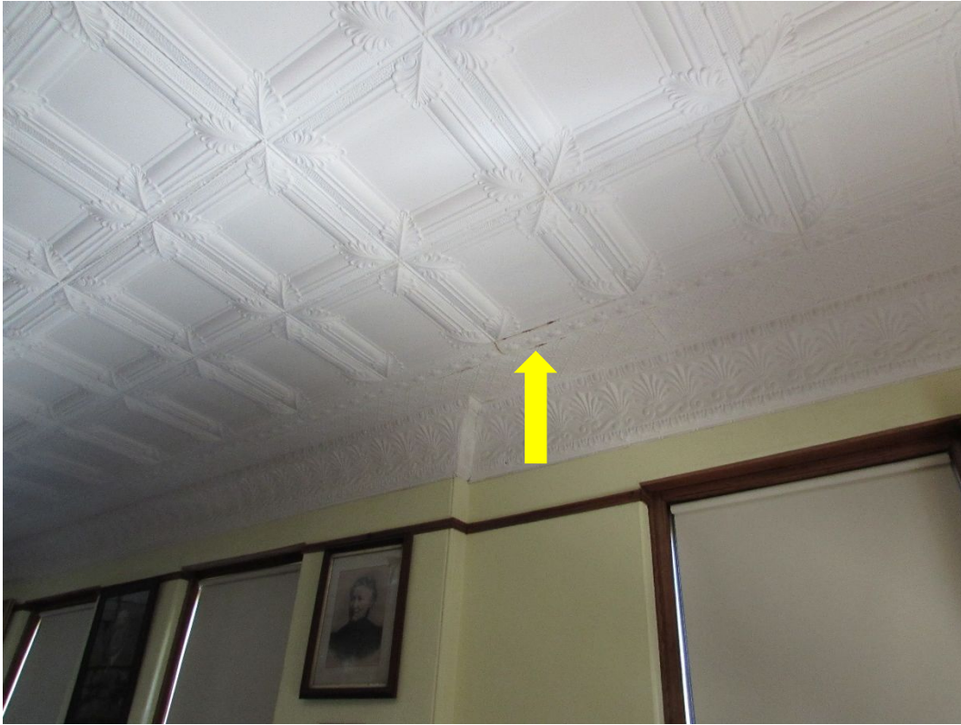
Photo #66 – Evidence of corrosion and water infiltration
