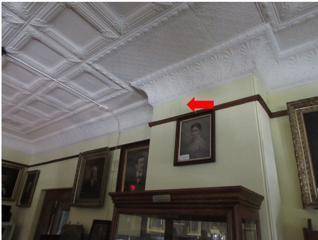
Photo #68 – Evidence of water infiltration at right sidewall of original structure
