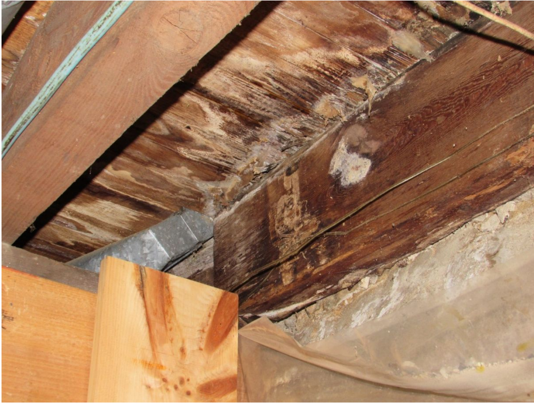
Photo #37 – Decayed joist and flooring along front wall
