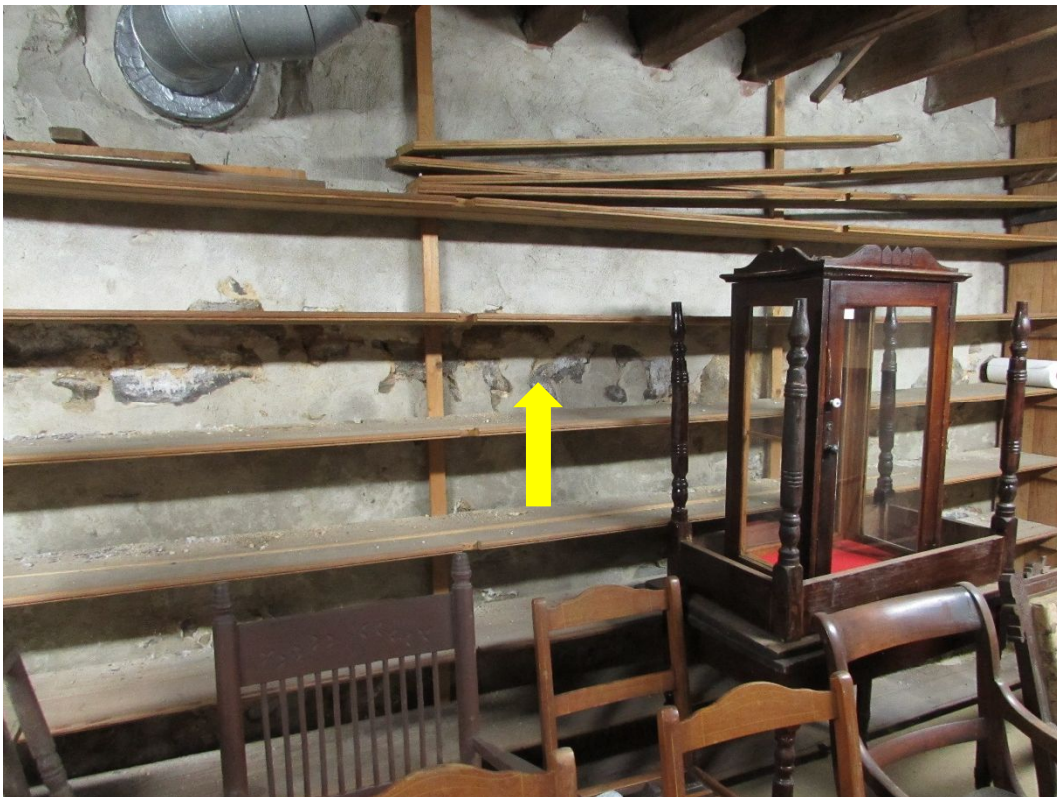
Photo #3- Loose spalled stucco finish on left foundation wall
