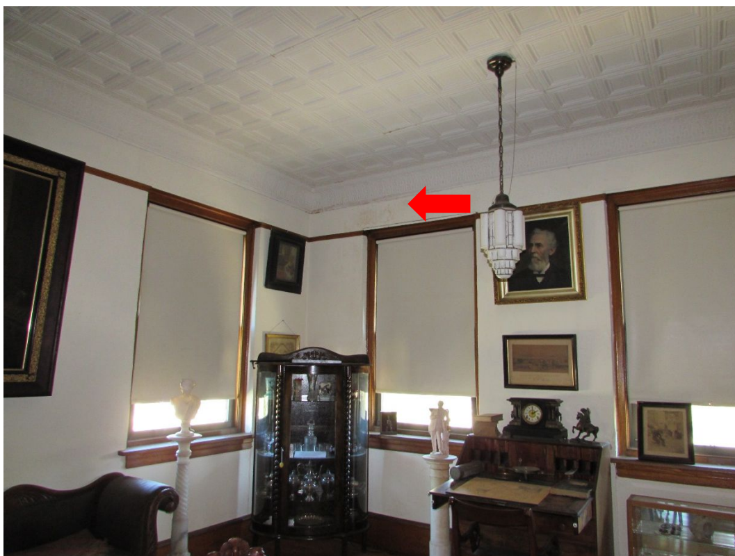
Photo #69 – Evidence of water infiltration at front right corner of 1933 addition
