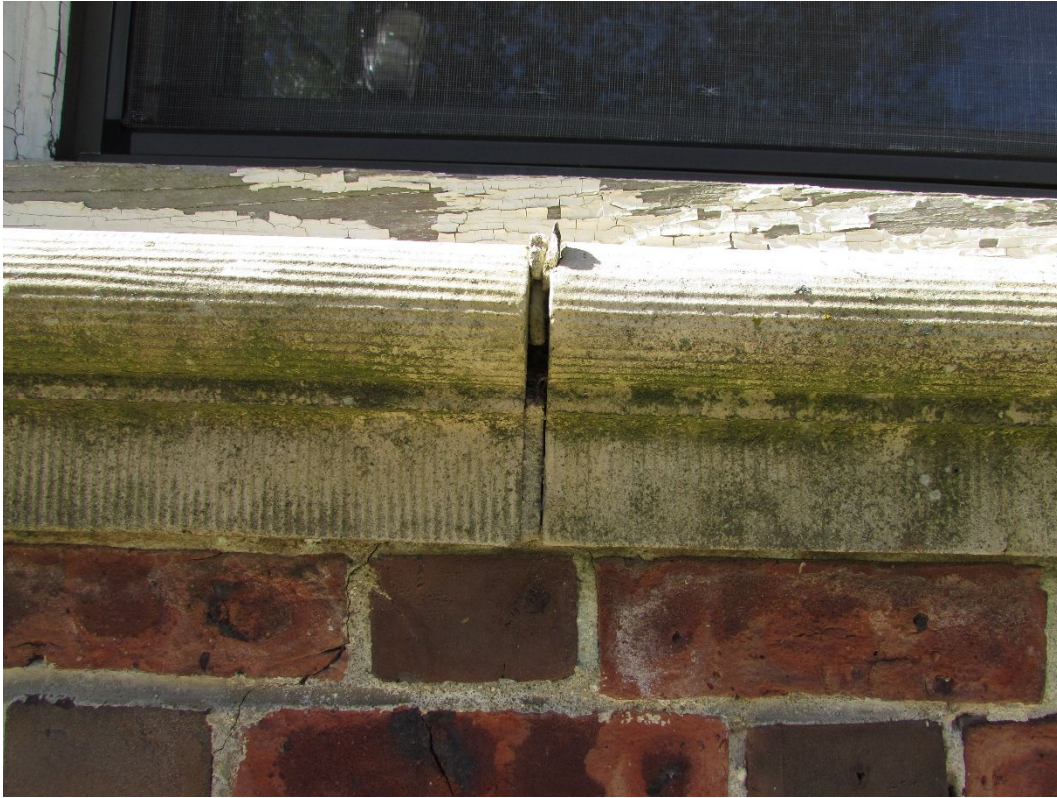
Photo #98 – Open Joint at precast window sill
