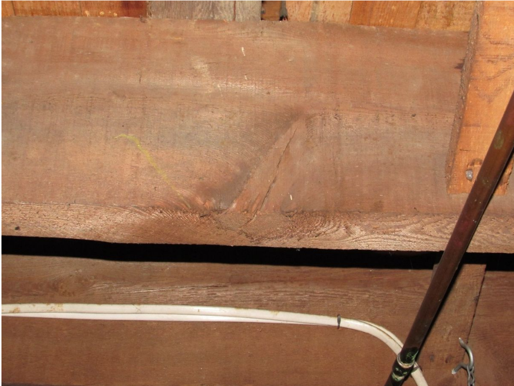
Photo #36 – Joist cracked at natural knot
