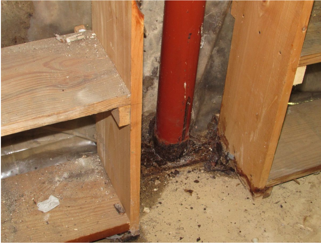
Photo #26 – Corroded base of column depicted in photo #25 above
