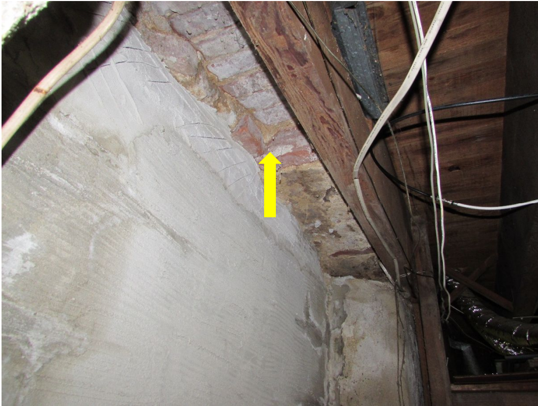
Photo #11 – Unsupported brickwork at infilled window opening
