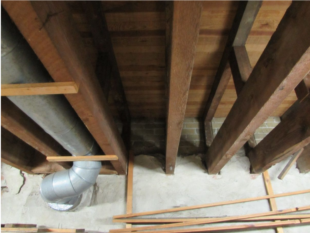
Photo #34 – Floor joists embedded in left sidewall
