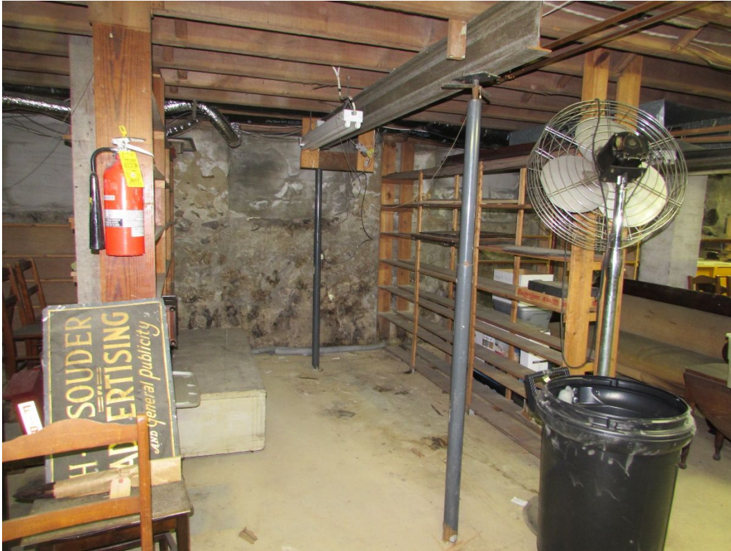
Photo #24 – Supplemental steel lally columns
