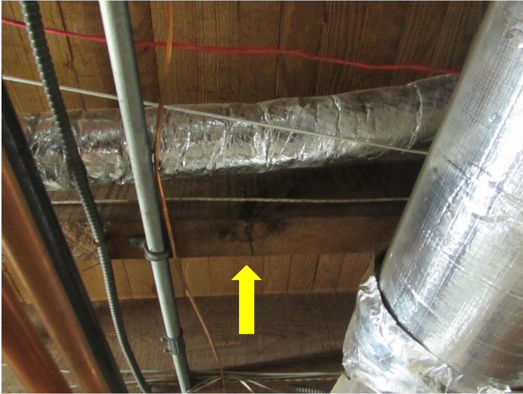
Photo #41 – Cracked flor joist
