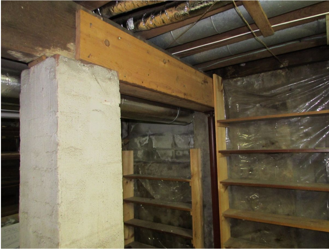
Photo #29 – Decayed girder reinforced by new lumber
