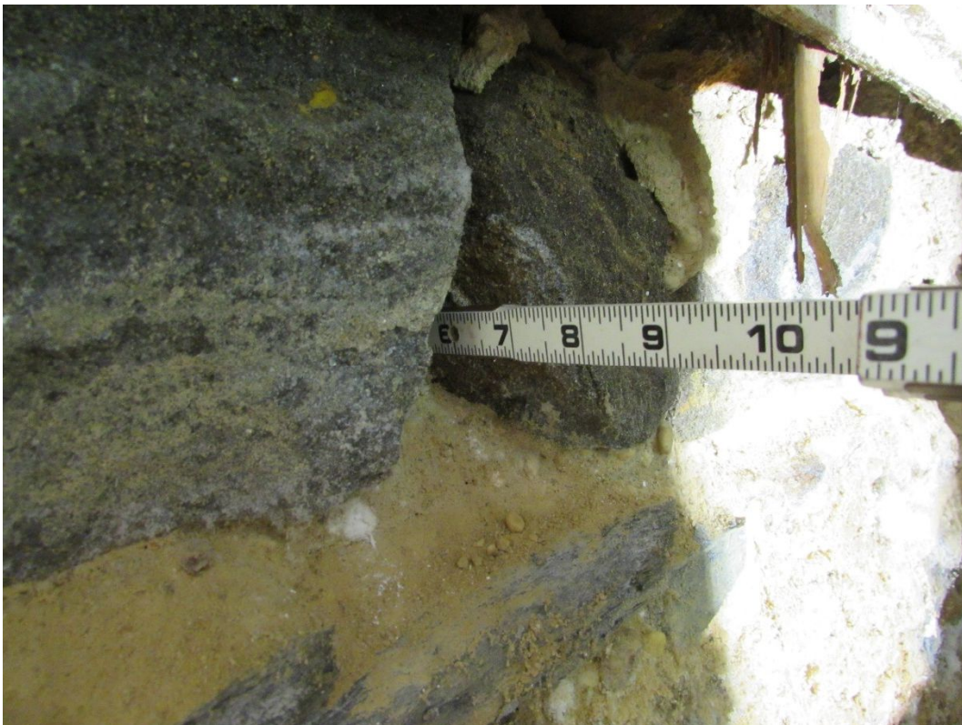
Photo #7 – Eroded mortar joint in photo #6 above
