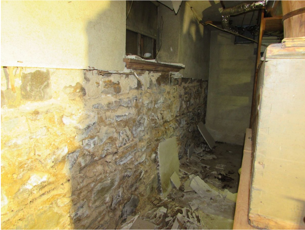
Photo #6 – Deteriorated rear left foundation wall
