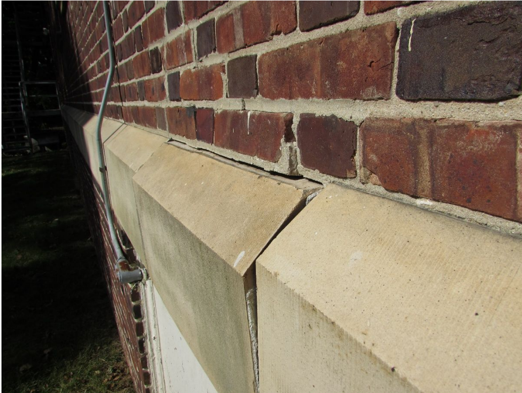
Photo #101 – Side view depicting movement of segment
