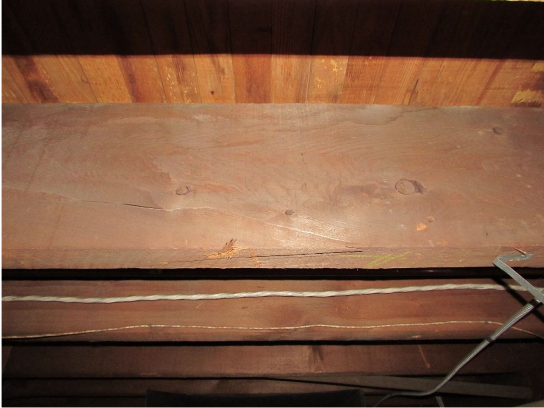
Photo #39 – Cracked floor joist in photo #38
