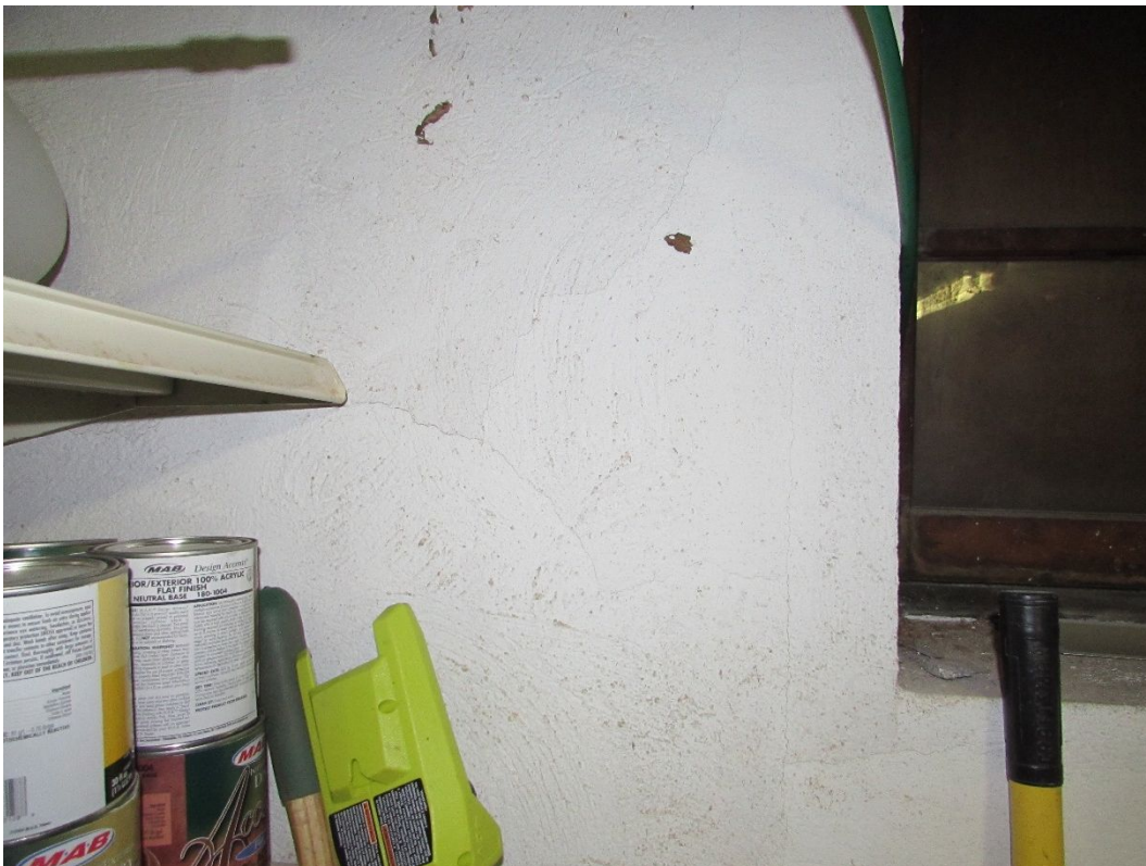
Photo #15 – Minor random hairline cracks in exterior workshop foundation wall
