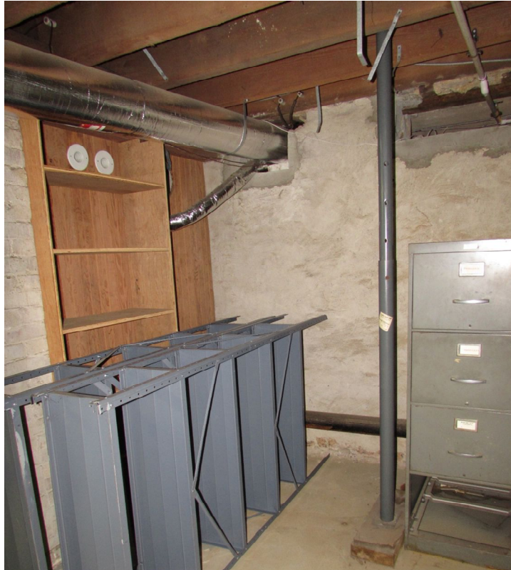
Photo #27 – Column beneath first floor safe
