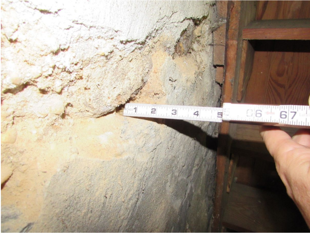
Photo #4 – Loose deteriorated mortar
