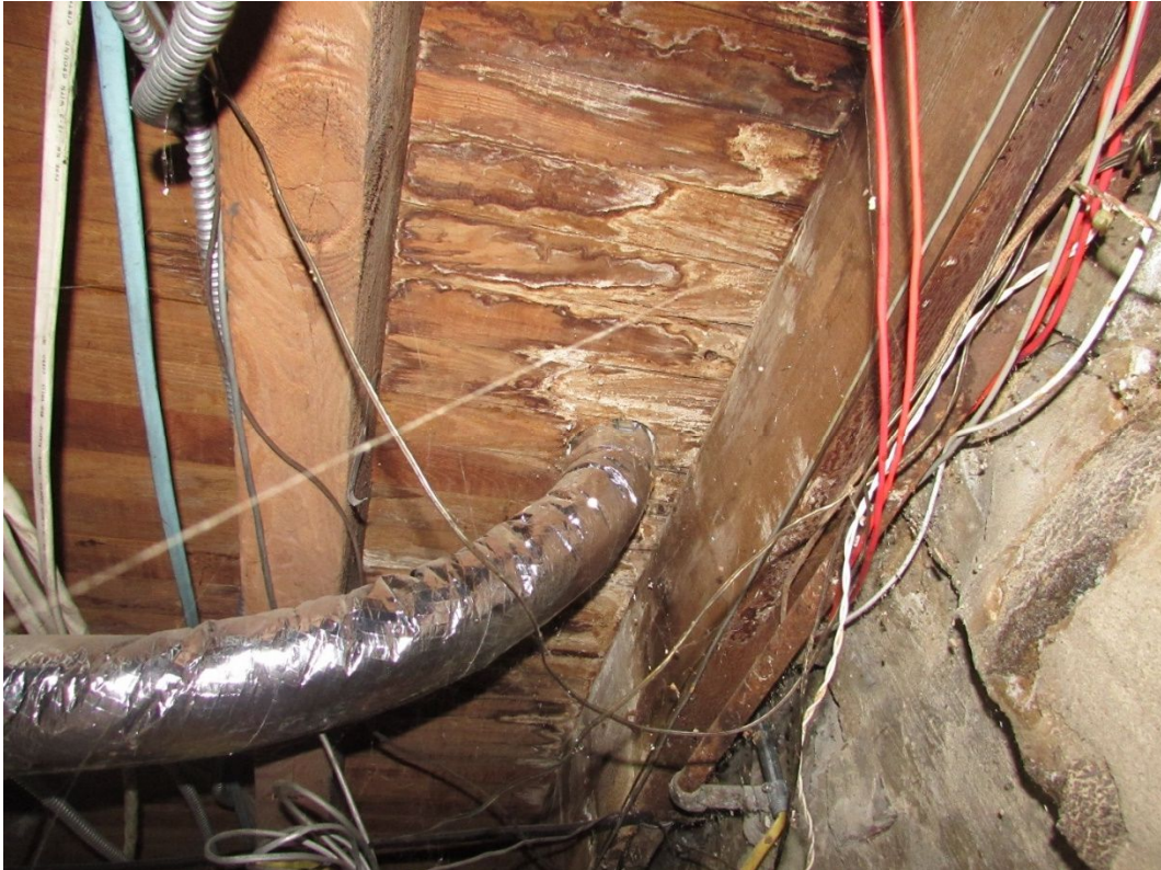
Photo #40 – Decayed flooring along front wall
