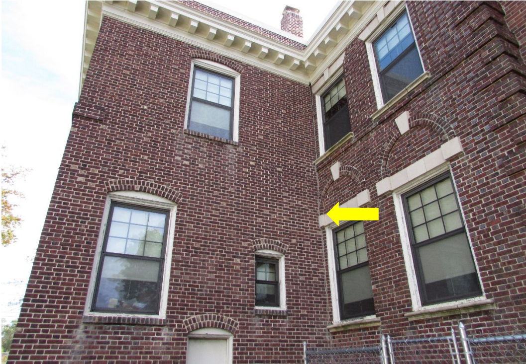
Photo #104 – Open joint (separation) of rear left corner of 1931 addition
