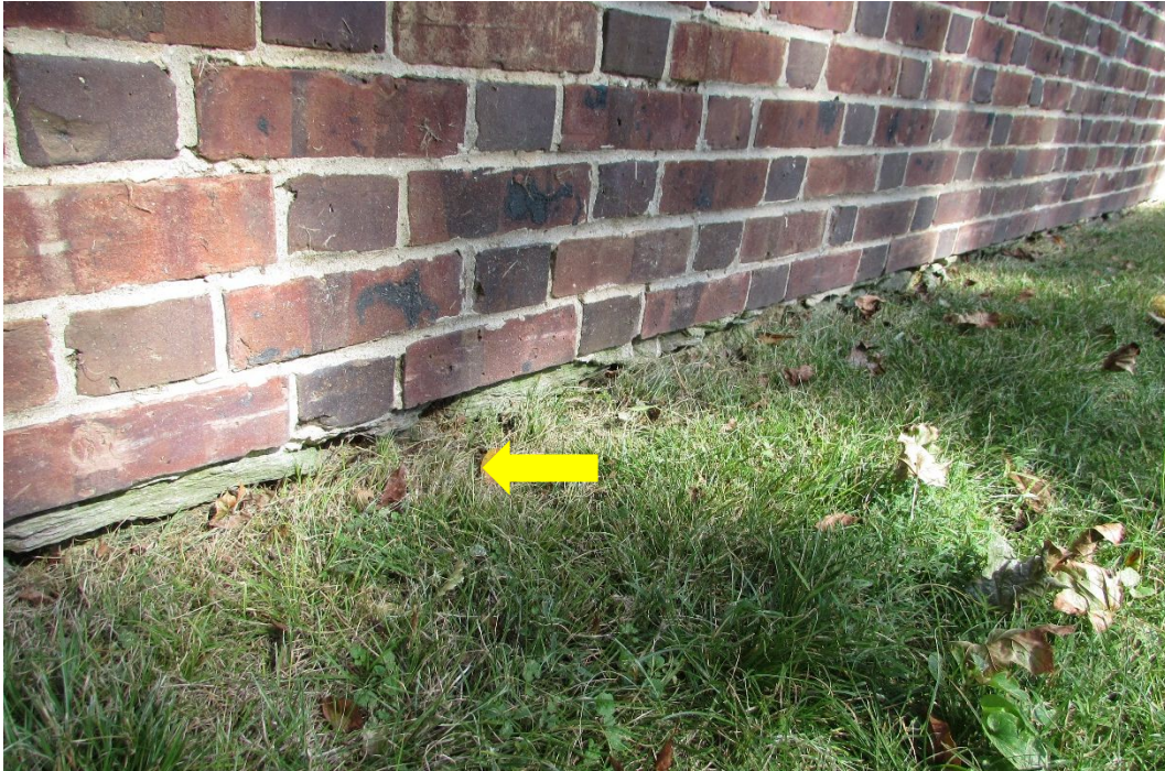
Photo #102 – Eroded joints of stone foundation wall
