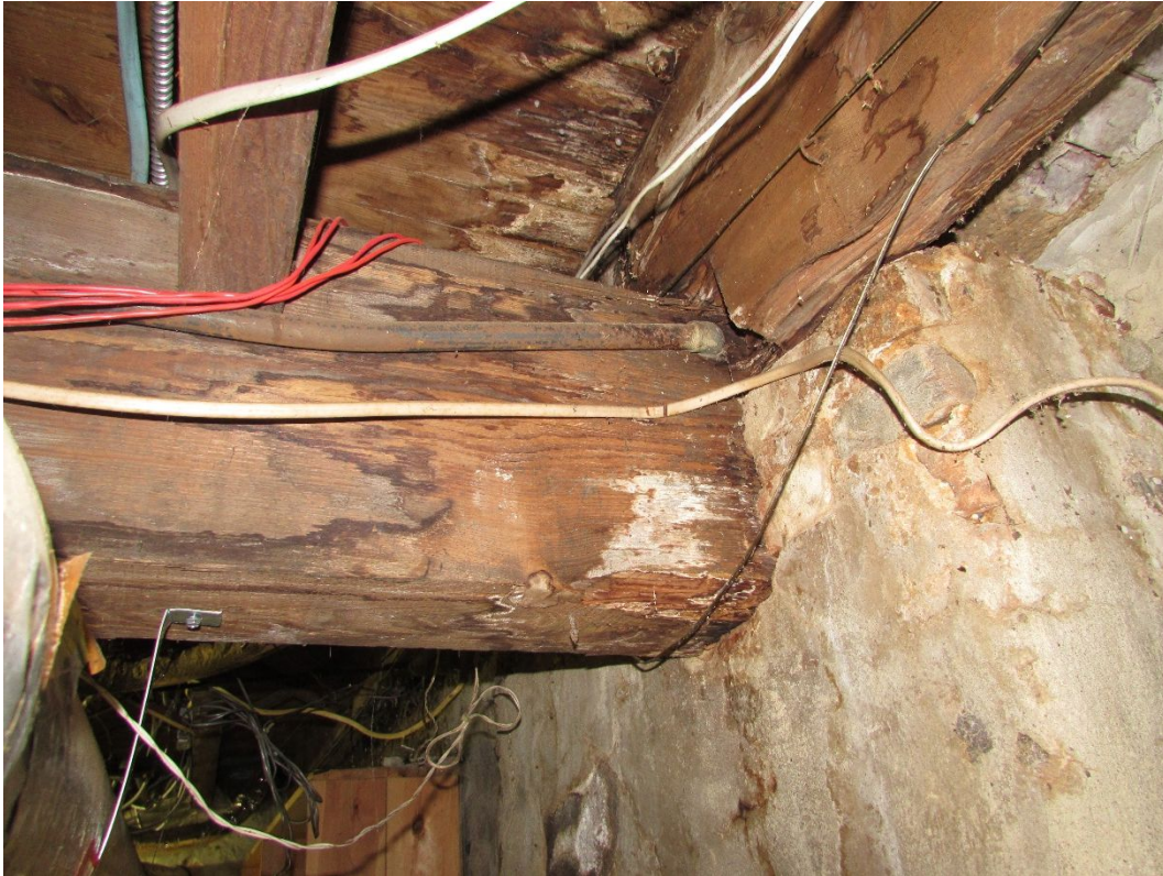
Photo #33 – Decayed girder and joist at front wall adjacent to right corner
