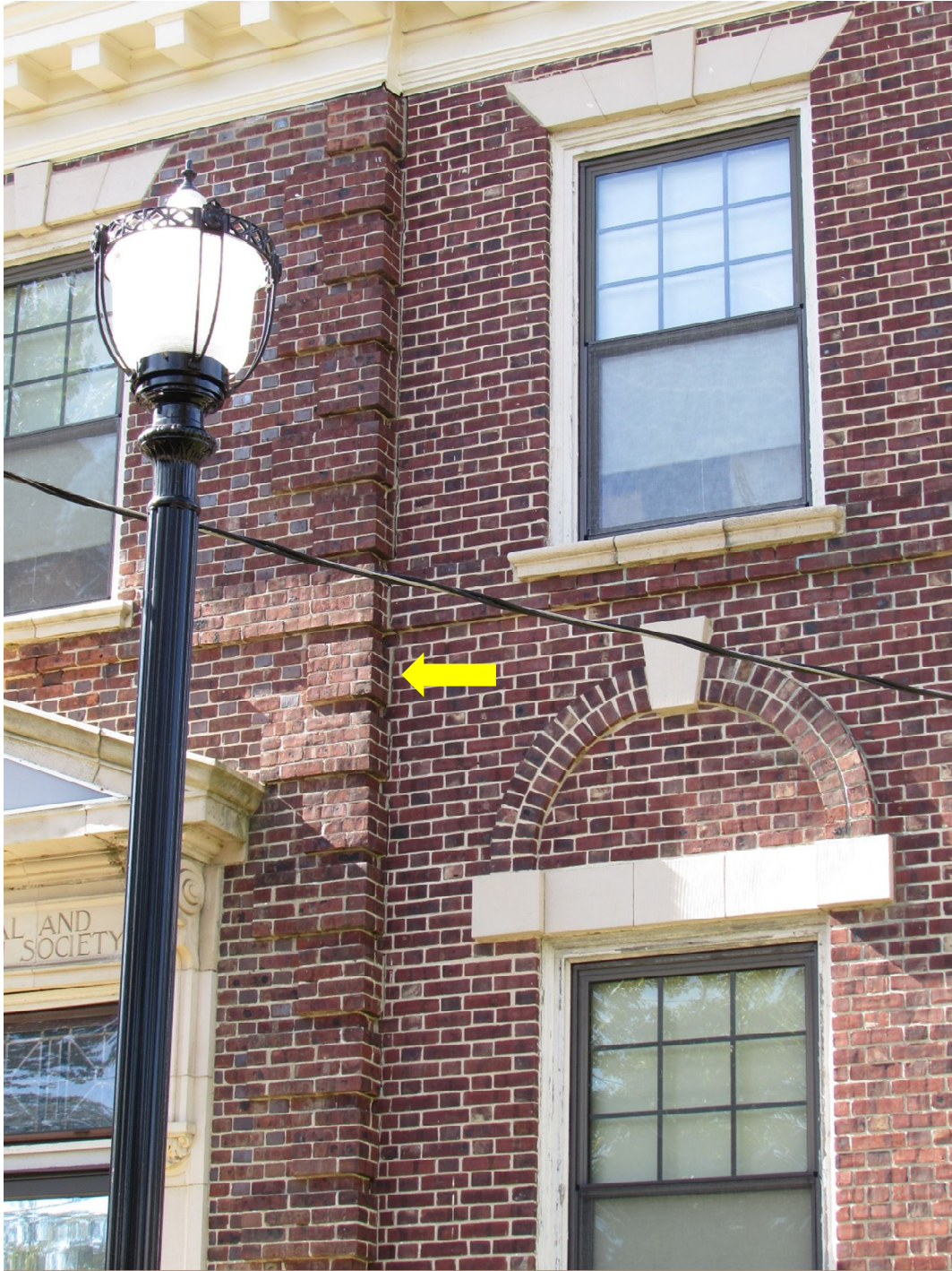
Photo #96 – Open joint between 1931 addition and original structure
