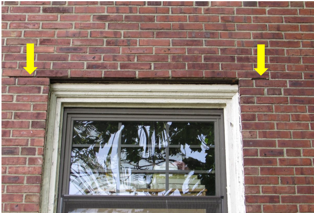
Photo #107 – Open joints at steel lintel
