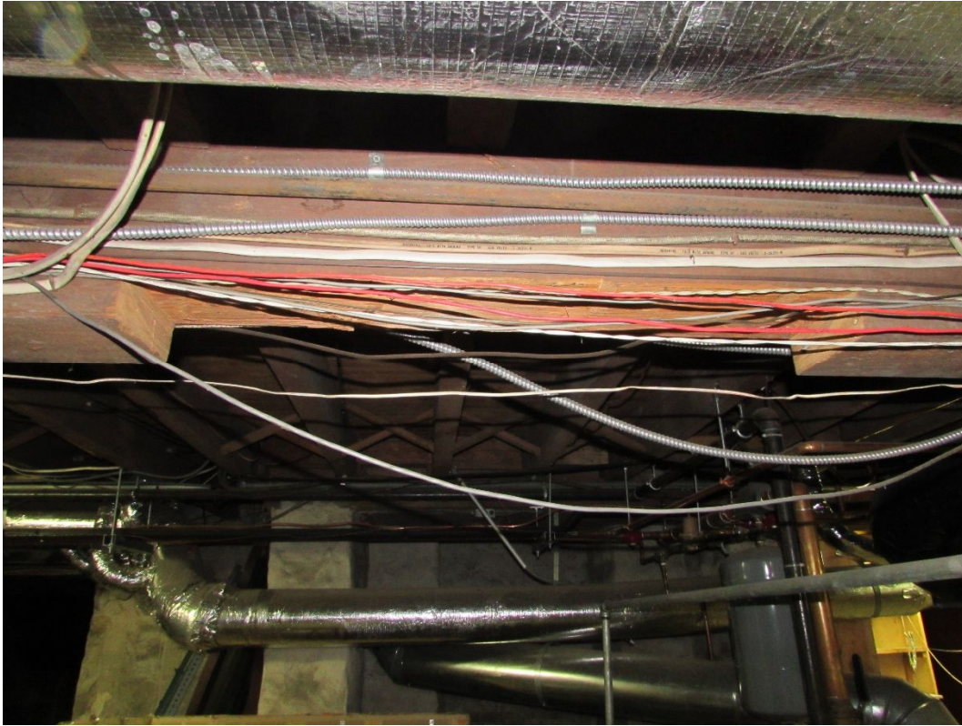
Photo #31 – Heavily notched girder
