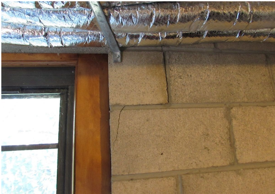
Photo #85 – Bearing crack at end of window header
