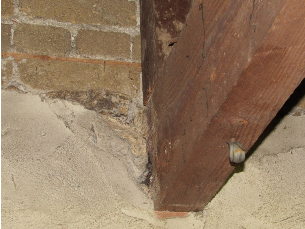
Photo #35 – Embedded joist end
