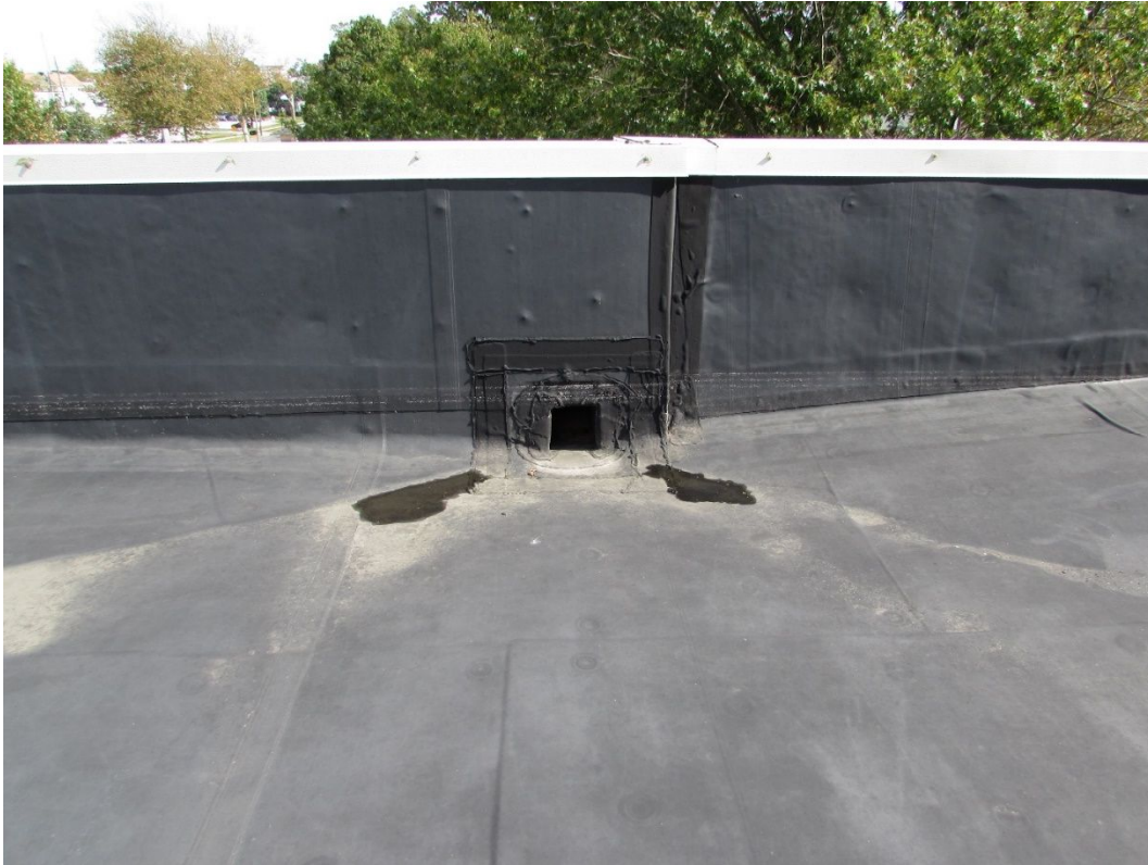
Photo #110 – Front roof scupper
