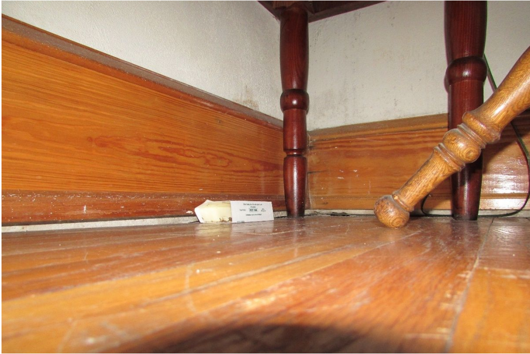
Photo #76 – Gap between wood floor and wall trim at Civil War Gallery
