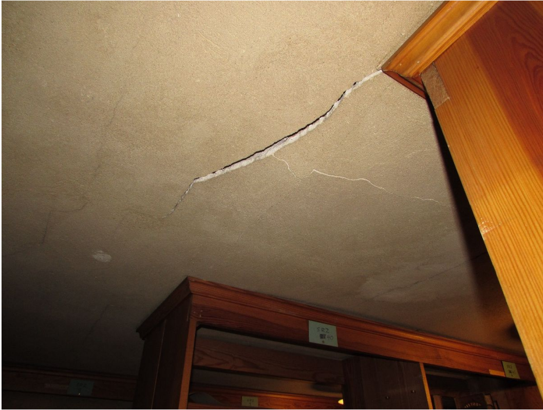
Photo #82 – Failing Plaster ceiling at Stack Room
