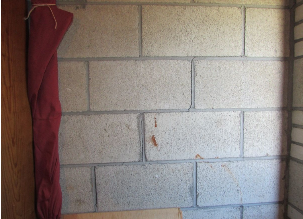
Photo #78 – Close up view of settlement cracking in photo #77 above
