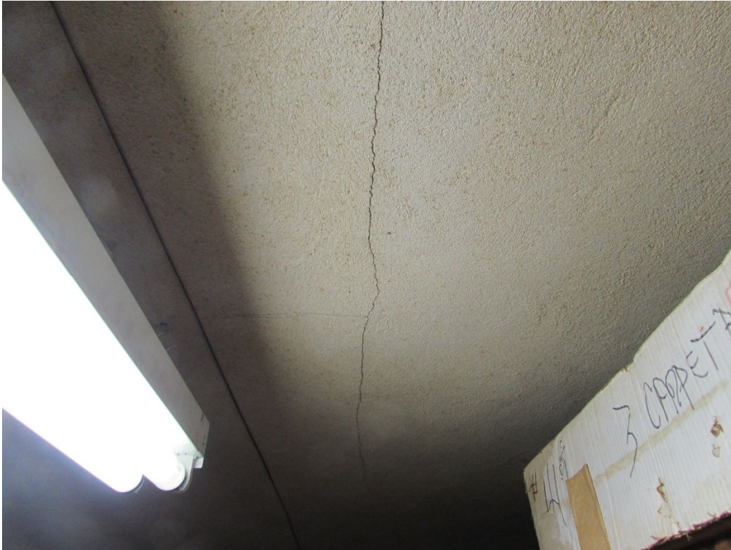
Photo #46 – Cracked plaster ceiling in photo #45 above
