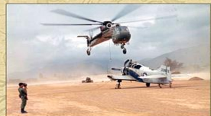
A CH-54 "Skycrane" (also known as "Flying Crane") lowers its hoist to recover a U.S. Air Force plane in Vietnam, circa 1966. (Courtesy of U.S. Army)
