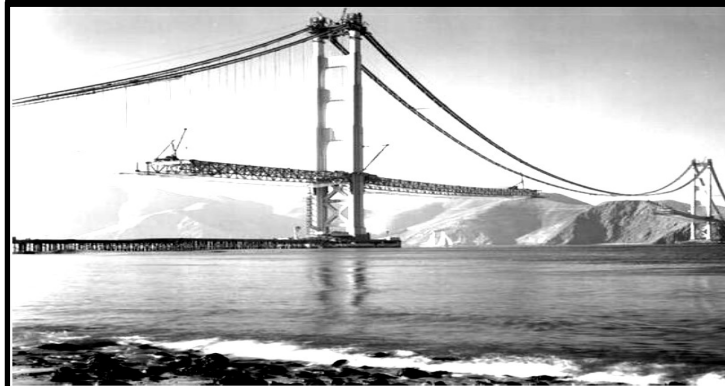
Golden Gate bridge construction, 1937
