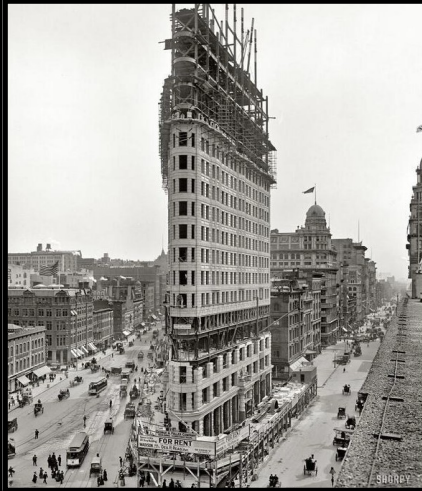
Flatiron Building, New York. The Manhattan landmark under construction. 1902
