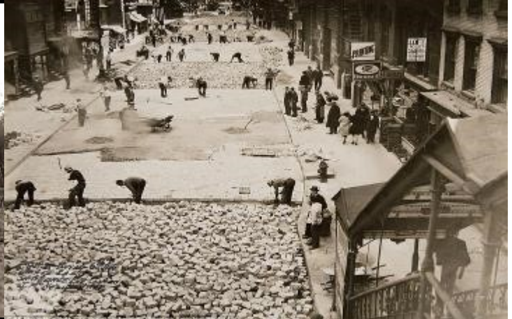
Laying a brick street in Manhattan in 1930
