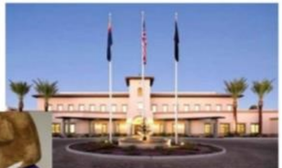
Above: Arizona State Veteran Home - Tucson
