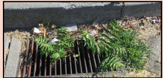
Tree of heaven growing in a storm drain
