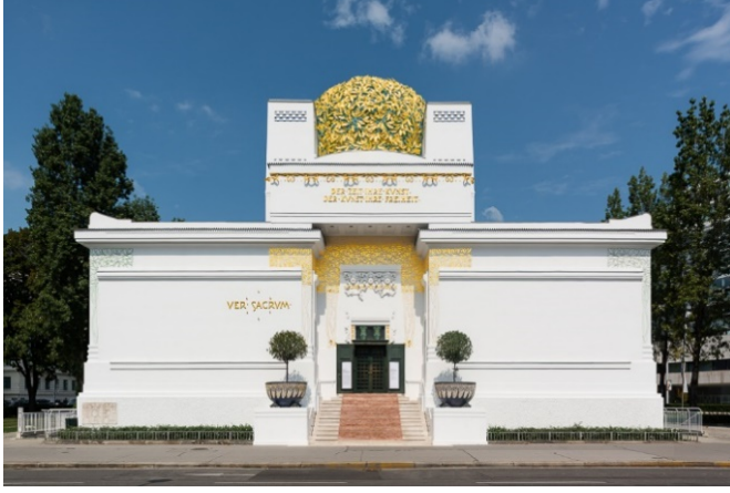
Figure 3. Front View of the Secession Building (Source: Secession, n.d.)
