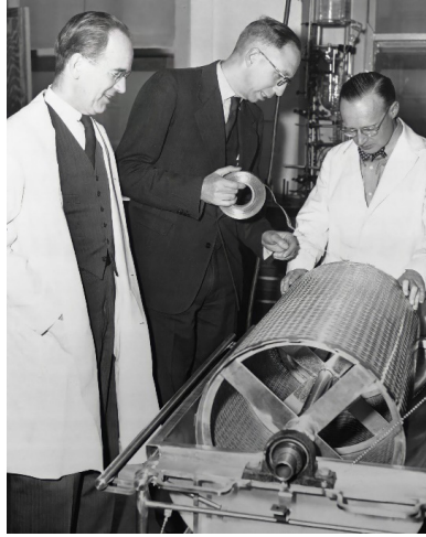
Figure 2. March 5, 1950: A cellophane tube containing human blood passes through a salt bath mixture in this new artificial kidney at Cleveland Clinic. Its developer, Dr. William J. Kolff, is the Dutch doctor who recently had joined the staff at the clinic. Looking on are Dr. Irvine H. Page, Research Director, and Dr. A. C. Corcoran, Asst. Research Director (Achievement, 2022).
