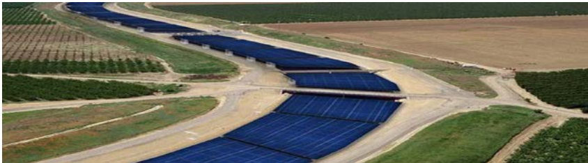
Fig. 3 Irrigation canals covered with solar PV panels.
