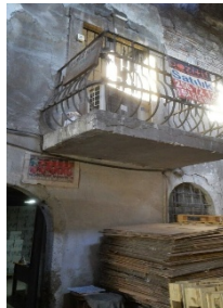
Picture 7. The balcony inside Çakaloğlu Han
