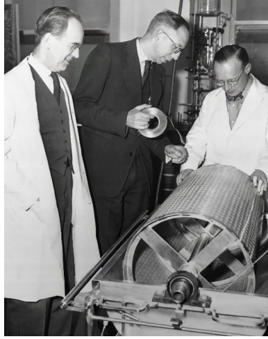
Figure 1. In 1947, Dr. Willem Kolff Designed the First Dialysis Machine (Kaempffert, 1947).
