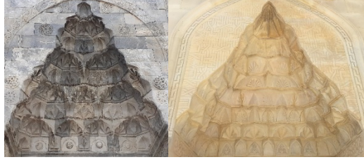
Figure 7. Aksaray Sultanhanı second portal muqarnas and Konya Ecdad Park portal muqarnas
