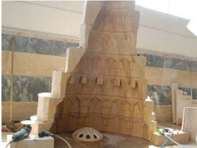
g) Placing muqarnas layers on top of each other
