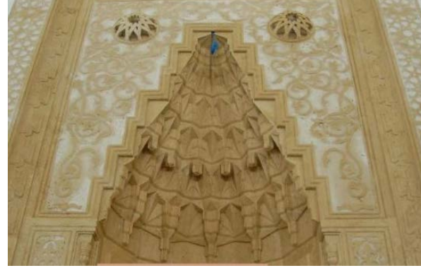
j) Completed mihrab muqarnas
