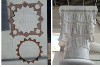
Figure 4. a. Steel sheet column capital molds, b. Column capital muqarnas
