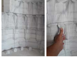
Figure 5. Placement of star units in muqarnas layers
