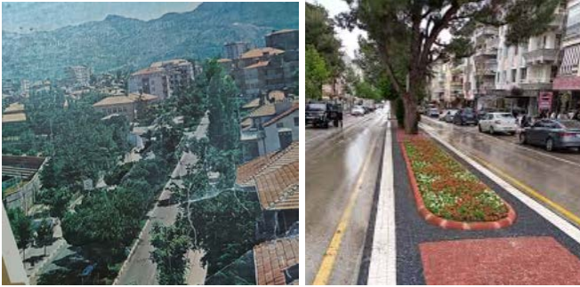
Figure 4. İstasyon Street in the 1980s (Turgut, 2000), İstasyon Street Today
