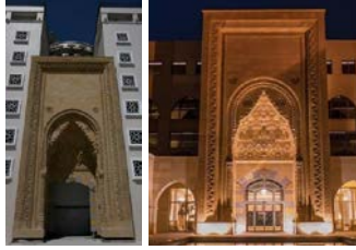
Figure 10. Distorted proportions of portal elements
