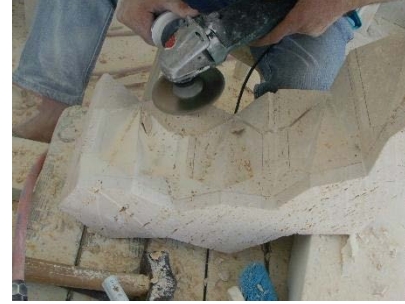
f) Final touches with cutting wheel
