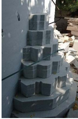
i) Backside of the muqarnas layers
