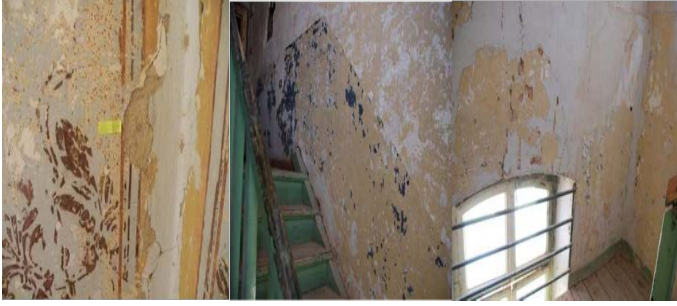
Figure 5. Ma'an Station Material Analysis and Restoration Report (Source: Gema Art International, 2012)
