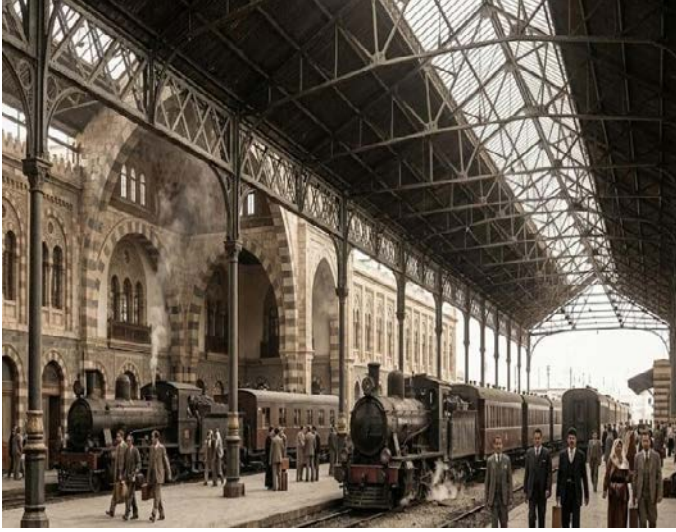
Figure 4. Sham Hijaz Station Roof Truss and Wide Span Tensioners ( https://www.diyanehaber.com.tr/foto-galeri/devrik-baas-rejimi-osmanli-yadigari-hicaz-demir-yolundaki-kadem-istasyonunu-harabeye-cevirdi(04.03.2026 – 21:33) )
