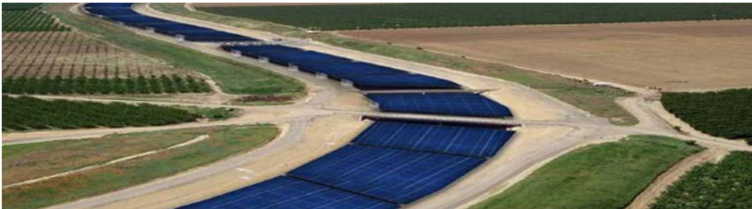
Fig. 3 Irrigation canals covered with solar PV panels.
