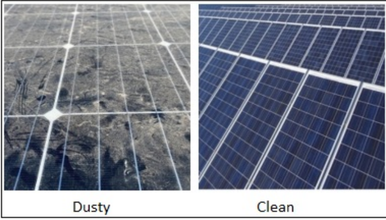
Figure 1. Example images of photovoltaic (PV) panels illustrating clean and dusty conditions used for CNN-based classification (adapted from Nogay, 2024a).
