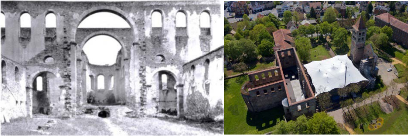
Figure 9. Bad Hersfeld Monastery after Restoration
