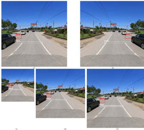
Figure 21. The results of the customized YOLOv8l model with transfer learning, TTA applied on a sample from RDD2022 dataset: (a) The result obtained with the original image (b) The result obtained with the image symmetrically mirrored from left to right (c) The result obtained with the image adjusted to 50% of the original resolution (d) The result obtained with the image adjusted to 75% of the original resolution (e) The result obtained with the image adjusted to 90% of the original resolution
