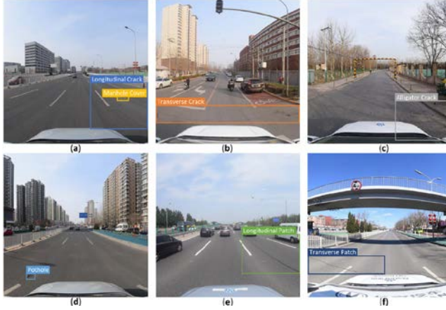
Figure 2. Sample images in the SVRDD dataset: (a) Longitudinal crack and manhole cover, (b) Transverse crack, (c) Alligator crack, (d) Pothole, (e) Longitudinal patch, (f) Transverse patch (Ren, Zhang, Zhi, Wei, & Feng, 2024)
