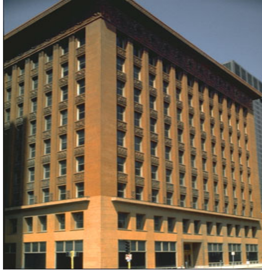
Figure 1. The Wainwright Building
