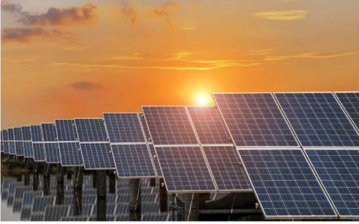
Fig. 1 An array of solar panels convert sunlight to electricity
