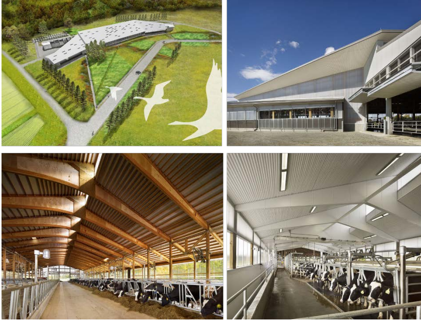
Figure 2. Example of roof designs in sustainable livestock facilities (Teaching Dairy Barn) (Erdy McHenry Architecture, 2022)
