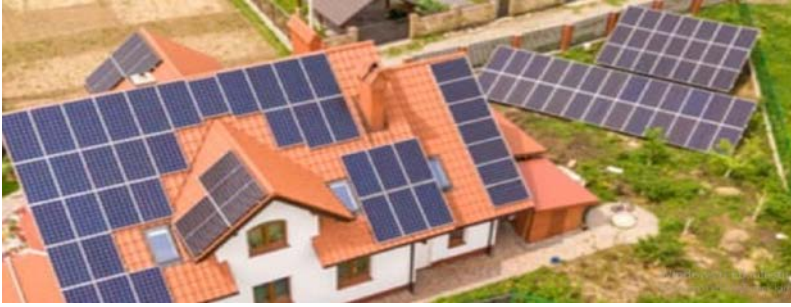
Fig. 4. A grid-connected rooftop solar PV system installed on a residential house
