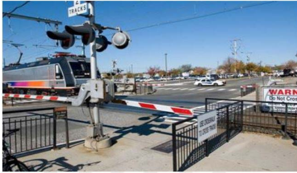
Figure 3.4. Example of a level crossing with barrier and automatic control (Bozlioğlu 2017)
