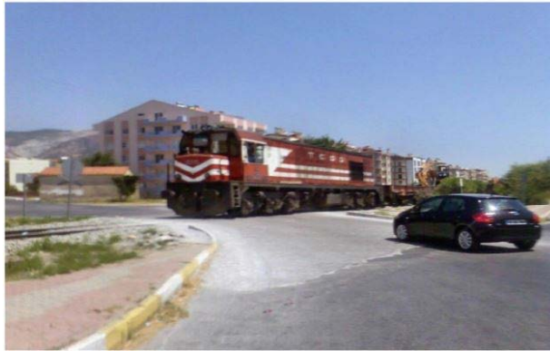
Figure 3.2. Example of an at-grade crossing without barriers and without a guard (completely uncontrolled) – 2 (Bozlioğlu 2017)
