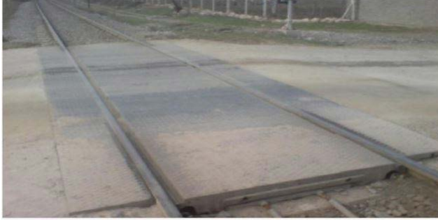
Figure 4.6. Rubber-coated level crossing (TCDD 2010)
