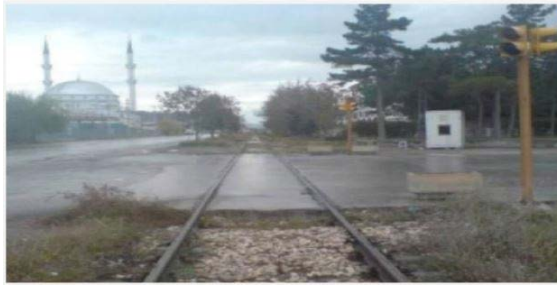
Figure 4.4. At-grade crossing with concrete-prefabricated pavement (TCDD 2010)
