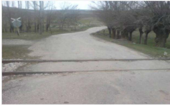
Figure 4.5. Asphalt-paved level crossing (TCDD 2010)
