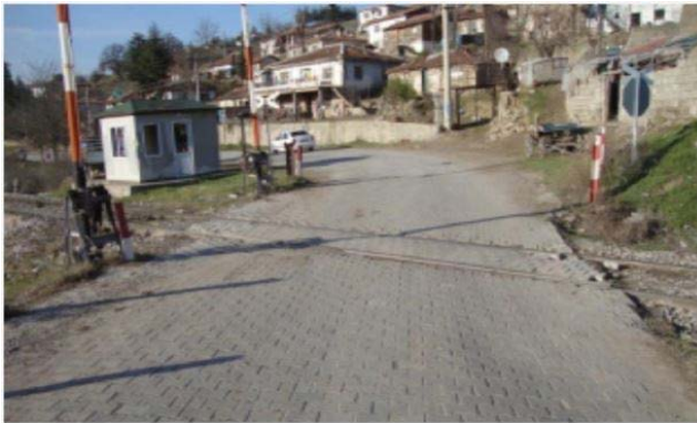
Figure 4.7. At-grade crossing with cut-stone pavement (TCDD 2010)
