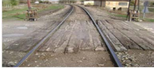
Figure 4.3. Wooden sleeper-covered level crossing (TCDD 2010)
