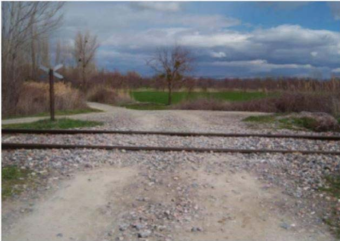
Figure 4.1. Ballast-gravel surface level crossing (TCDD 2010)
