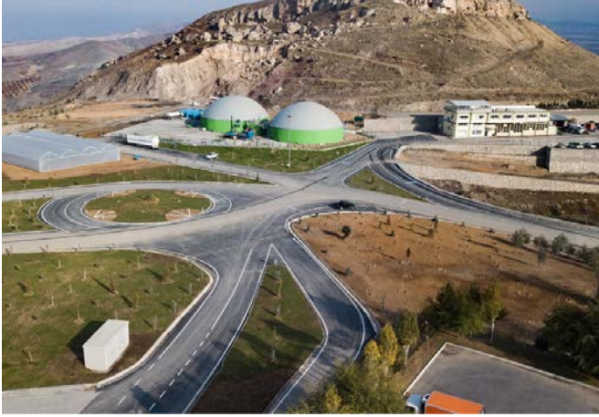
Figure 11. Malatya Landfill Gas Power Plant (Anyenerji.com, 2017)
