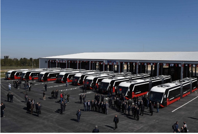
Figure 12. Malatya Trambus Vehicles and Maintenance Building (Ditemyapi.com, 2023)
