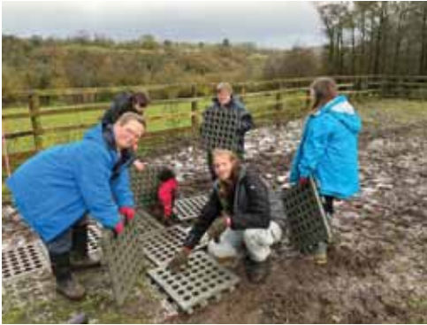
Busy volunteers helping lay mudcontrol slabs.
