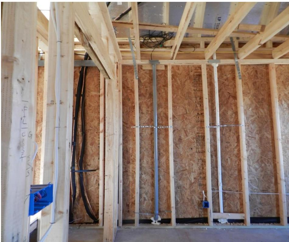
In this photo, the dark gray PVC pipe conveys coax from the attic to an antenna outside the house. Note the coil of coax near the top of the pipe. This coil will be routed down an interior wall and into the new ham shack.
