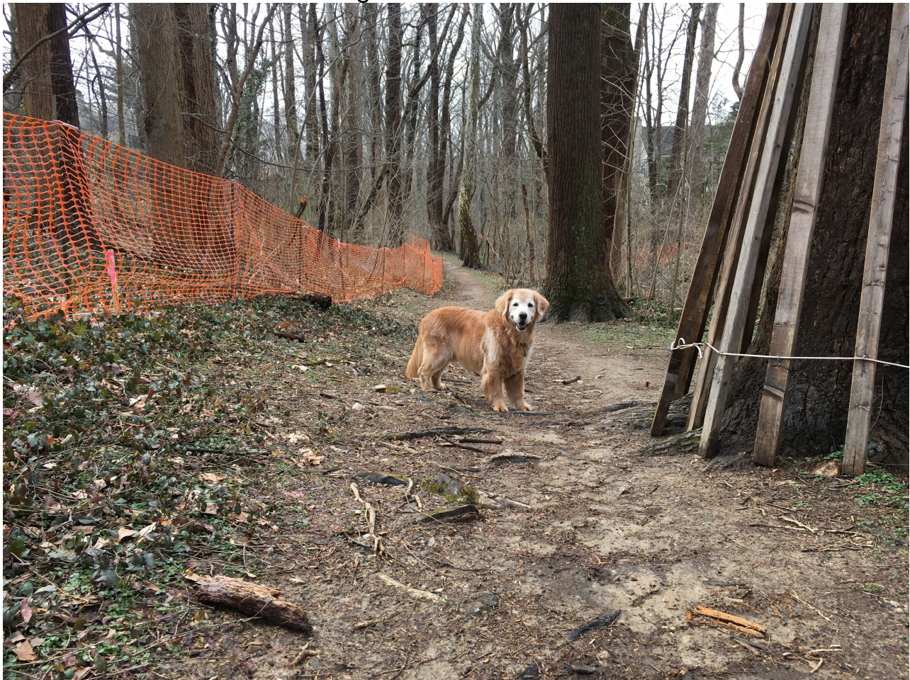
Quincy, one of the neighborhood's most frequent users, explores the construction in Spring Valley Park that will restore the walking trails that have badly eroded.
