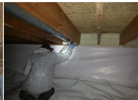
A crawl space with adequate drainage will still have moisture problems, coming from two major sources: the **ground** and the **outside air**. Ground water will evaporate into a dirt-floored crawl space and soak the joists and wooden structures. It will also infiltrate concrete walls and floor causing them to be damp most of the time. It is not possible to effectively insulate a crawlspace without eliminating these major moisture sources.
