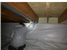
A crawl space with adequate drainage will still have moisture problems, coming from two major sources: the **ground** and the **outside air**. Ground water will evaporate into a dirt-floored crawl space and soak the joists and wooden structures. It will also infiltrate concrete walls and floor causing them to be damp most of the time. It is not possible to effectively insulate a crawlspace without eliminating these major moisture sources.
