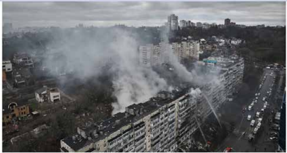
Drone view of a damaged building in the center of Kyiv as State Emergency Service provides assistance to the victims and puts out the fire on Jan. 2, 2024, in Kyiv, Ukraine. (Kostiantyn Liberov/Libkos/Getty Images)
