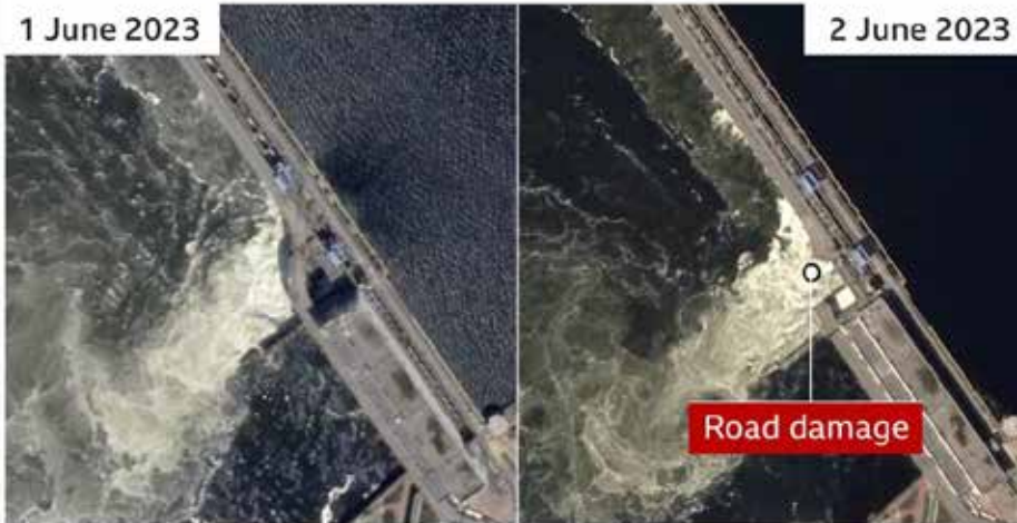
Satellite images show damage to roadway
