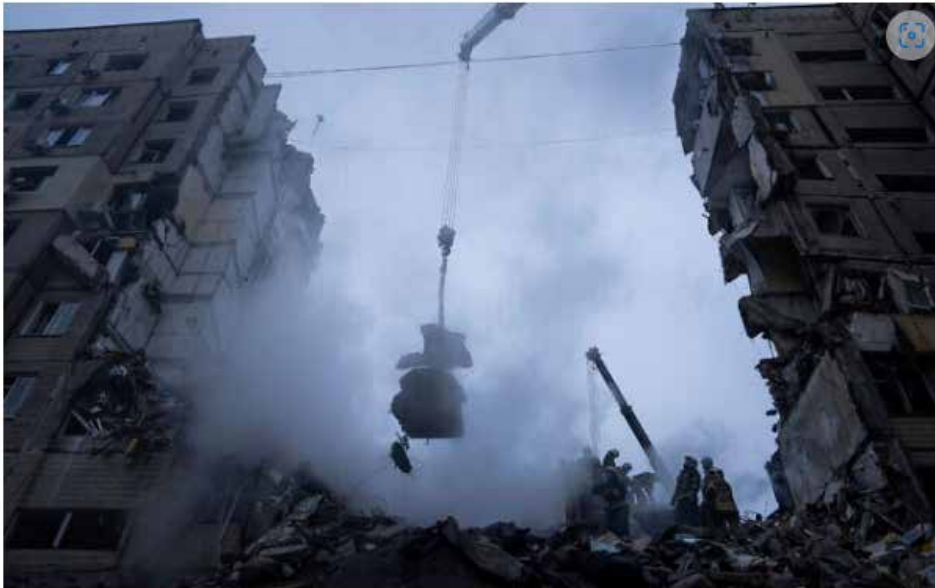
Rescue workers clear the rubble from an apartment building that was destroyed in a Russian rocket attack at a residential neighbourhood in the southeastern city of Dnipro, Ukraine, January 15, 2023. (AP Photo/Evgeniy Maloletka)
