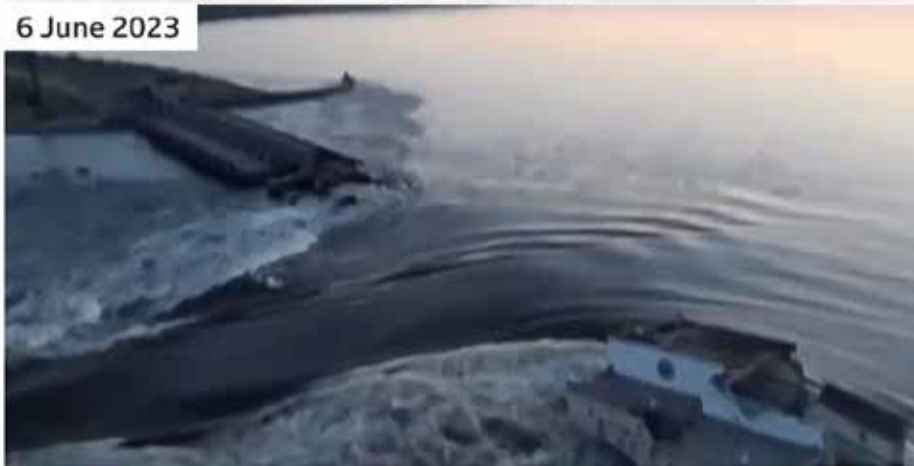
Aerial video shows breach of larger sections of the dam
