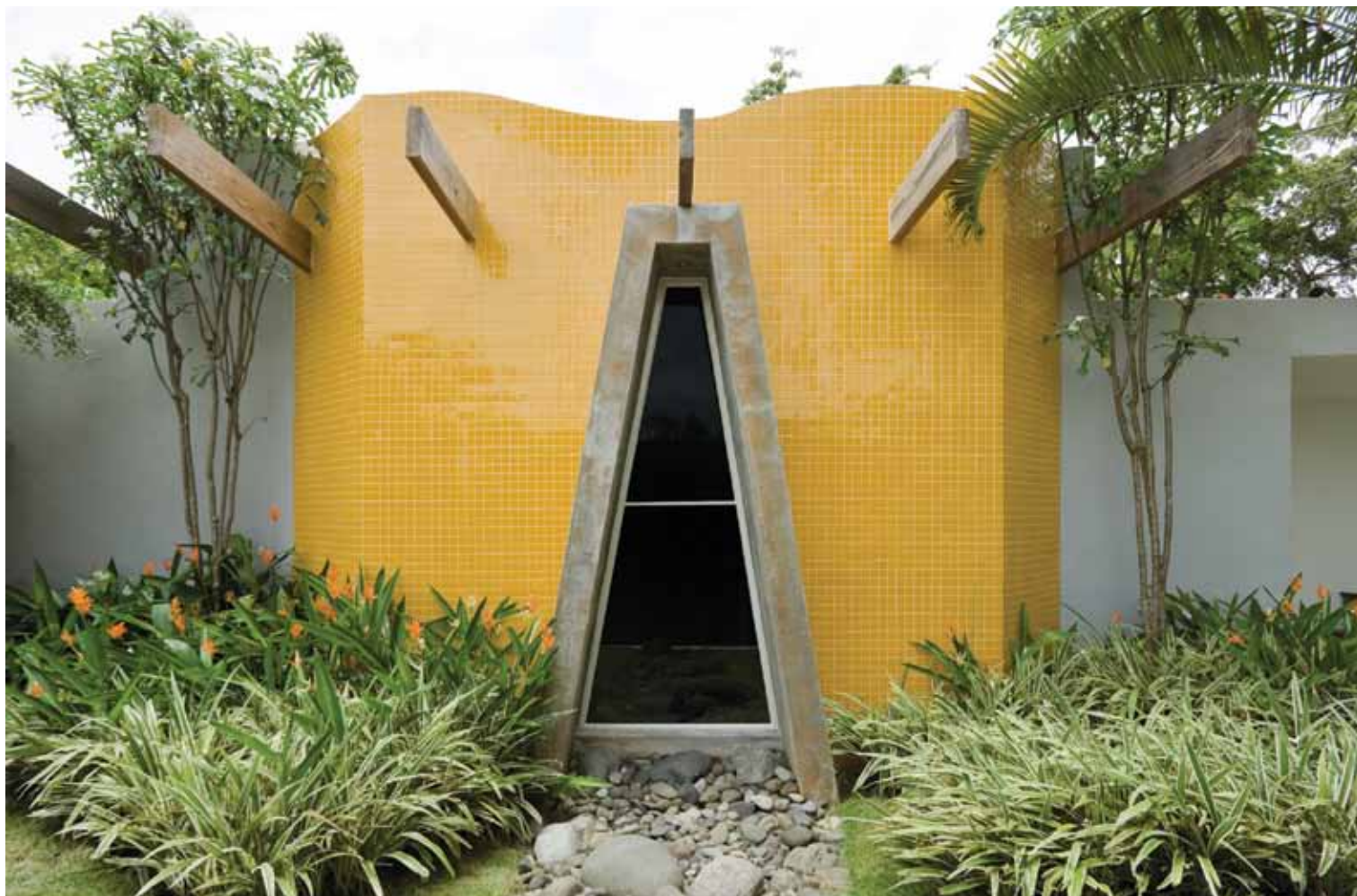
arte_FIST .FOUNDATION's offices at Dorado, Puerto Rico.
