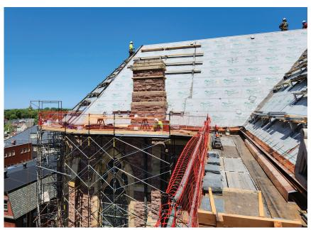
sure there are no cracks. The slate will ping in just the right way to confirm, soundness. In addition, slate was pulled from three separate pallets onto one, to maintain even color dispersion across the roof plane, to eliminate blotches of lighter and darker slates.
