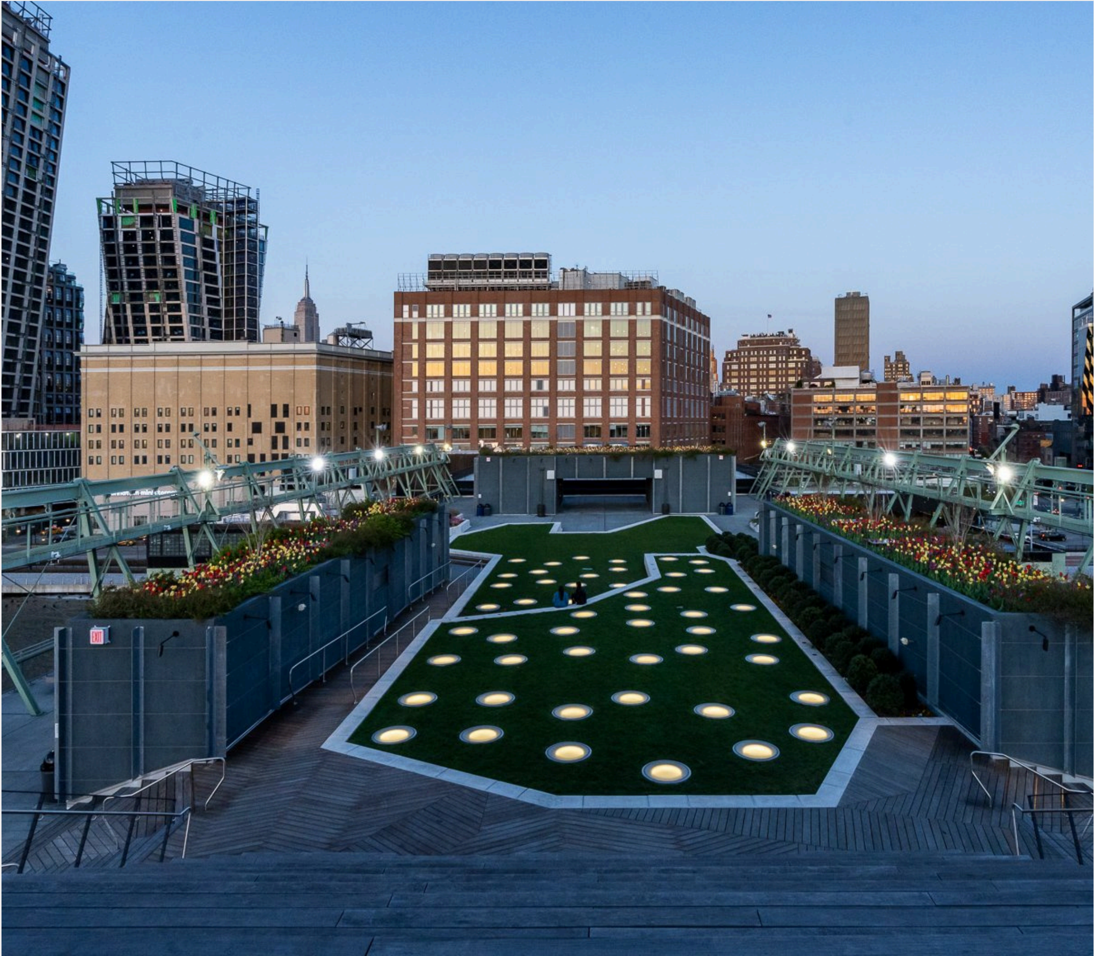
EACH SKYLIGHT TAPERS IN SECTION, ALLOWING FOR VARIOUS EXISTING STRUCTURAL, MECHANICAL AND PLUMBING CONDITIONS TO REMAIN, THIS CREATES AN ARTFUL PLAY OF LIGHT AND SHADOW THROUGHOUT THE DAY IN THE MAIN LOBBY SPACE BELOW. THE SKYLIGHTS INTERFACE WITH THE NEW ROOFTOP PARK, DESIGNED BY !MELK AND HANDEL ARCHITECTS
